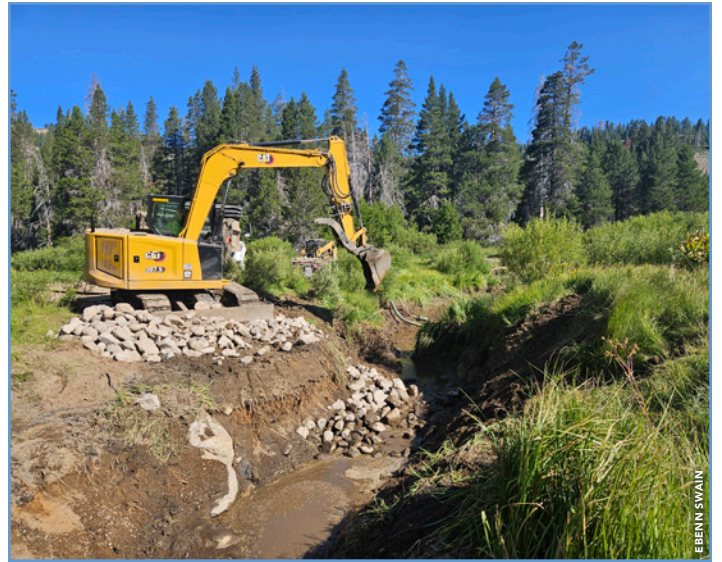
Rock weirs in the South Fork of Prosser Creek will prevent the stream from cutting deeper into the meadow surface, reducing erosion and sediment inputs during floods and big winters.
