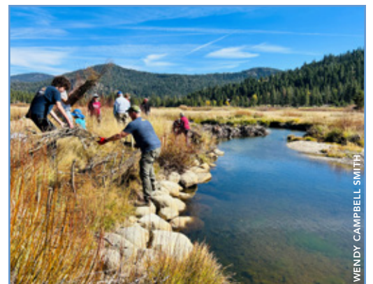
Volunteers at Truckee River Day! Bank stabilization along Washeshu Creek.
