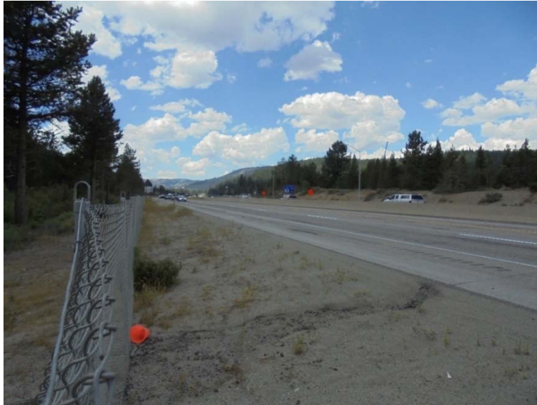
Figure 2. Site 4 rilling from freeway runoff, looking west; grass-lined swale with check dams proposed along south side (left) of fence.
