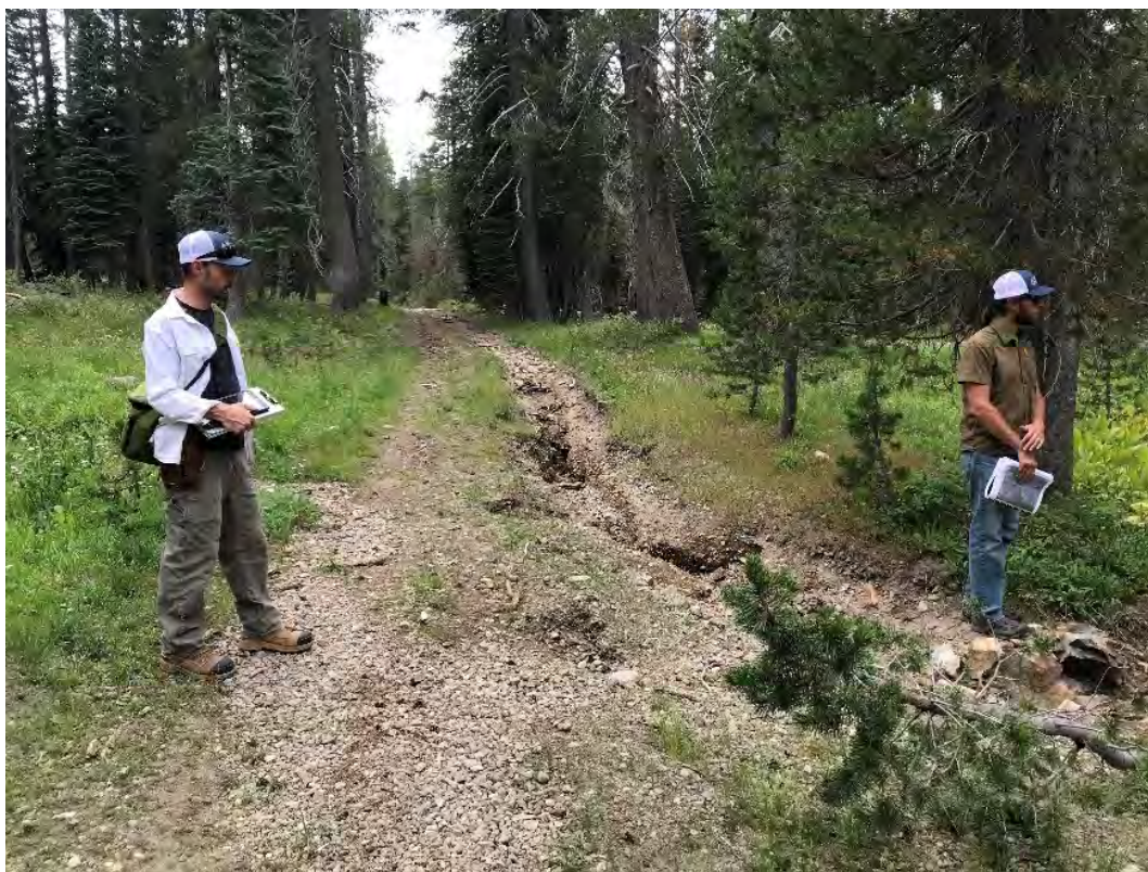
Figure 3-2 Example of Road Capture from Webber Lake Road.
