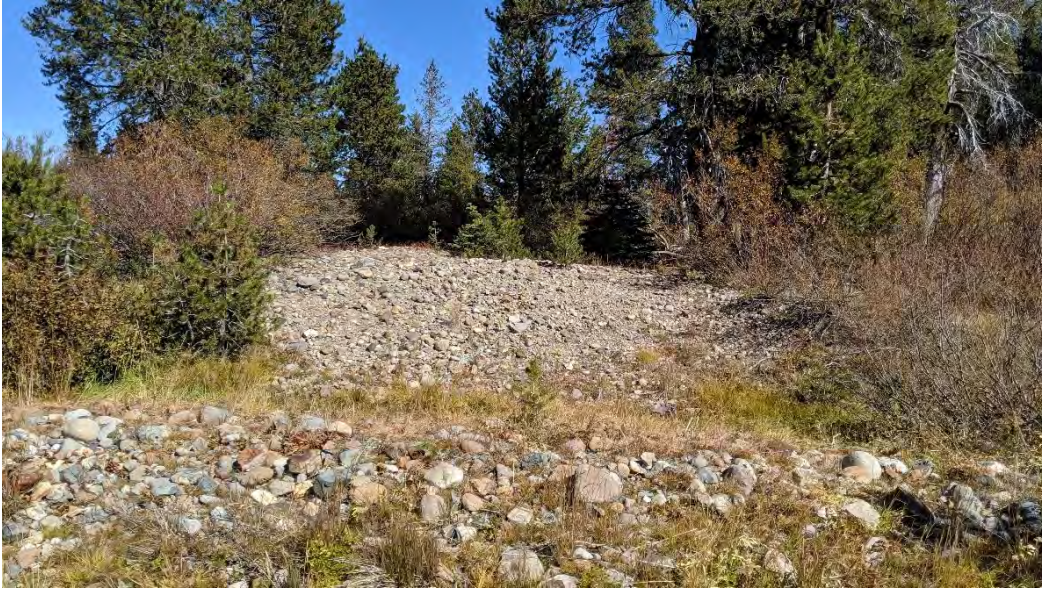
Figure 3-7 Former Main-Channel Blocked by a Push-up Dam, Lacey Creek, Upper Lacey Meadow. This dam encouraged channel avulsion to the northern side of the meadow and through the forest [Reach G(a)], depriving meadow of hydrologic support.
