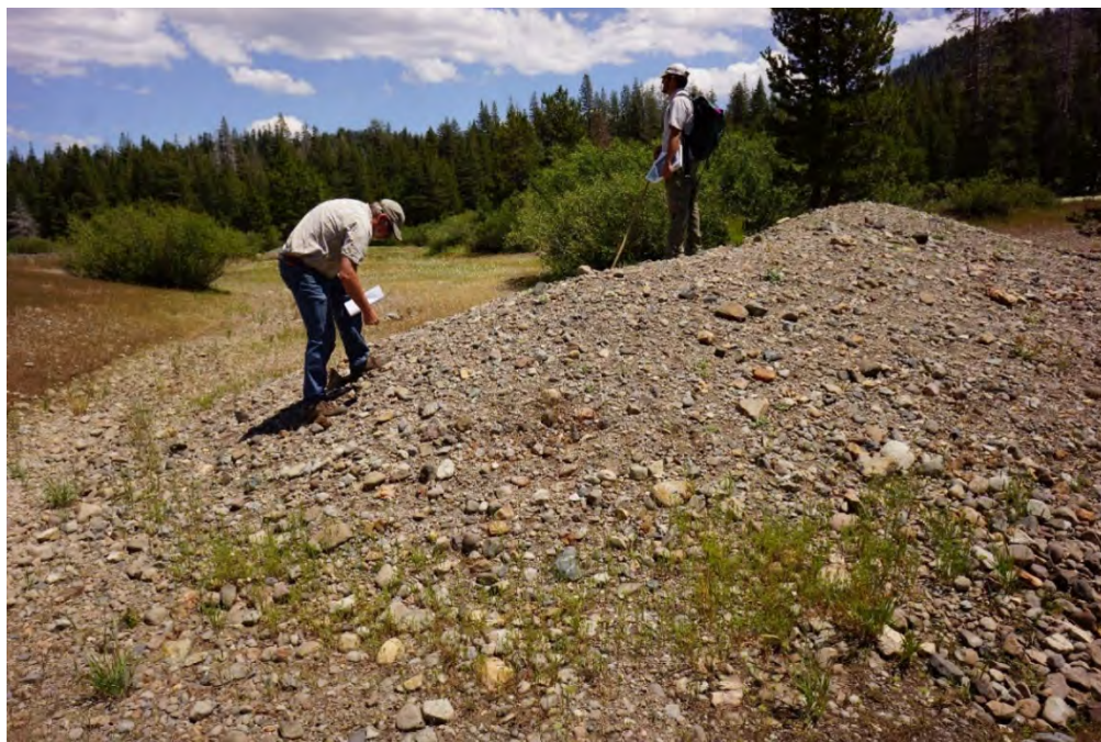
Figure 3-5 Example of a Gravel Push-up Dam Located in a Historical Channel of Lacey Creek, Upper Lacey Meadow, Reach G (b).
