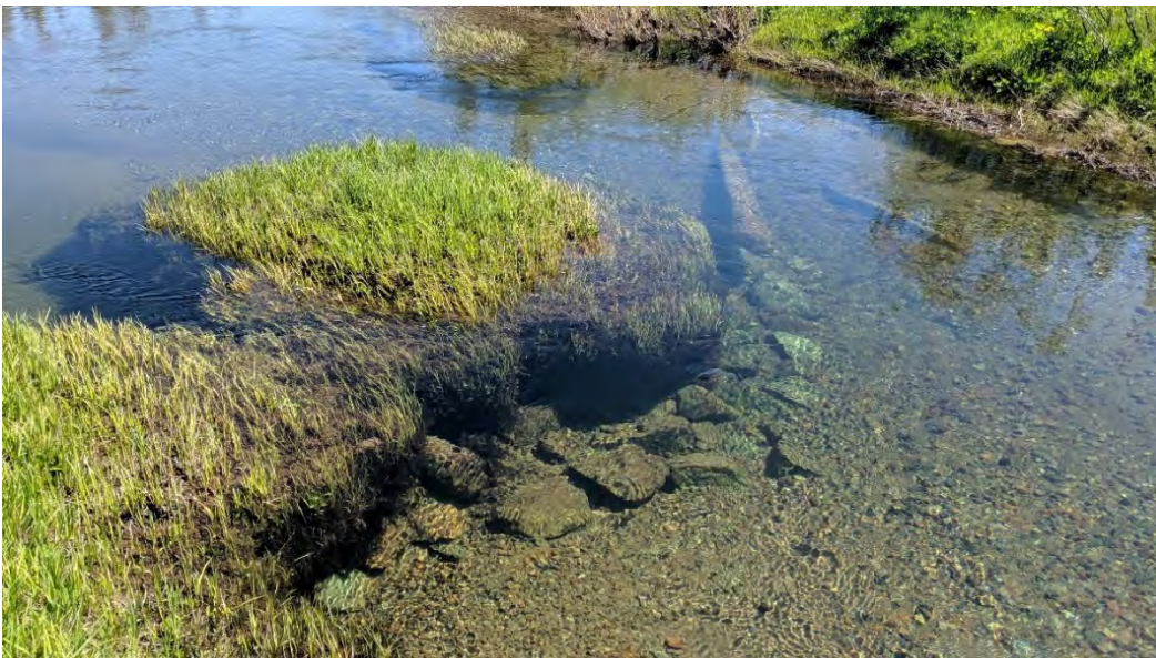
Figure 3-8 Example of an Old Rock and Log Dam or Diversion Structure, Lacey Creek, Lower Lacey Meadow, Reach B.
