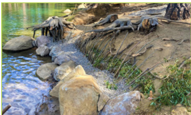
Bank stabilization using natural granite revetments and live willow plantings to prevent erosion and capture sediment.
