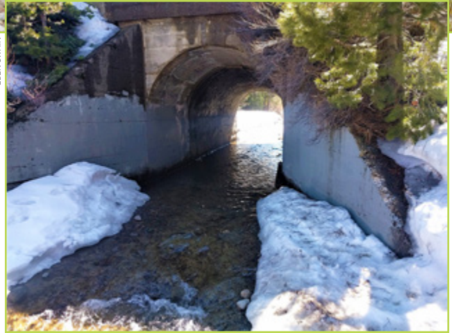
Railway tunnel channelization has resulted in high velocity flows and extreme erosion of streambanks downstream.
