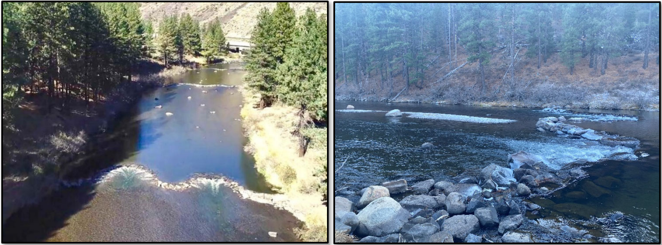
Figure 8. (Image left) Drone footage of series of three W-weirs looking upstream (Trout Unlimited). (Image right) Photo of W-weir taken from left bank looking S/W taken December 2020.
