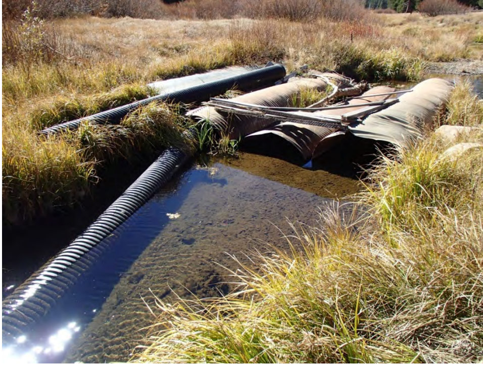
Figure 26. The culverts are filling with sediment and have created some widening at the stream margins
