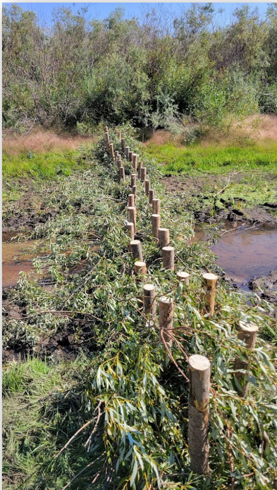
Example of "beaver dam analog" or BDA, Upper Truckee Marsh, South Lake Tahoe, CA, Balance Hydrologics, 2021
