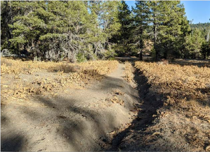
Road capture and gully erosion, former road and existing trail above corral
