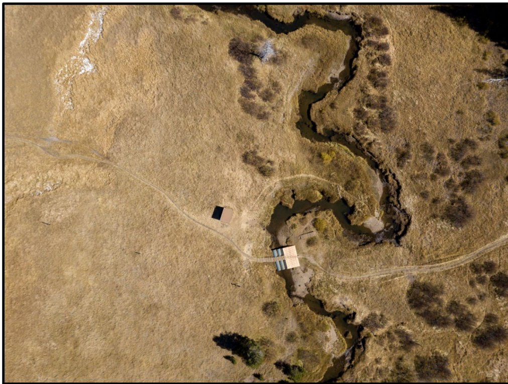
Figure 12. View of existing culverted crossing (Coyote Crossing). (Source: TDA Drone Footage)
