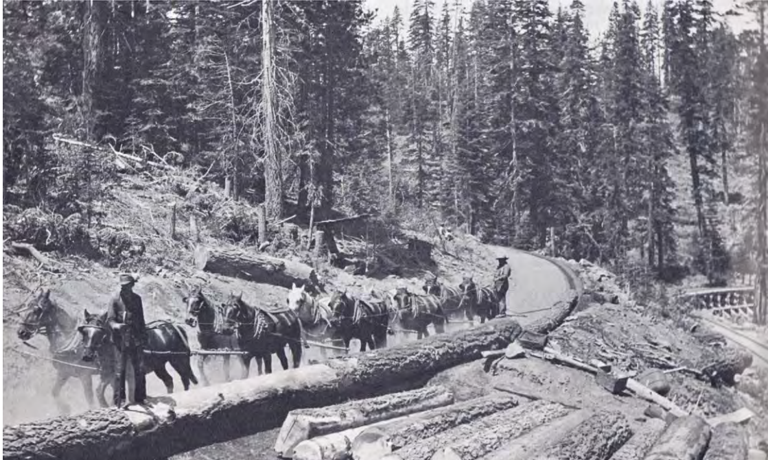
Photo 11. Horse teams were also used to skid timber in log chutes to inclined log decks, like this one along the Sierra Nevada Wood & Lumber Co.'s narrow gauge line (courtesy George D. Oliver Collection In Myrick 1962:444)
