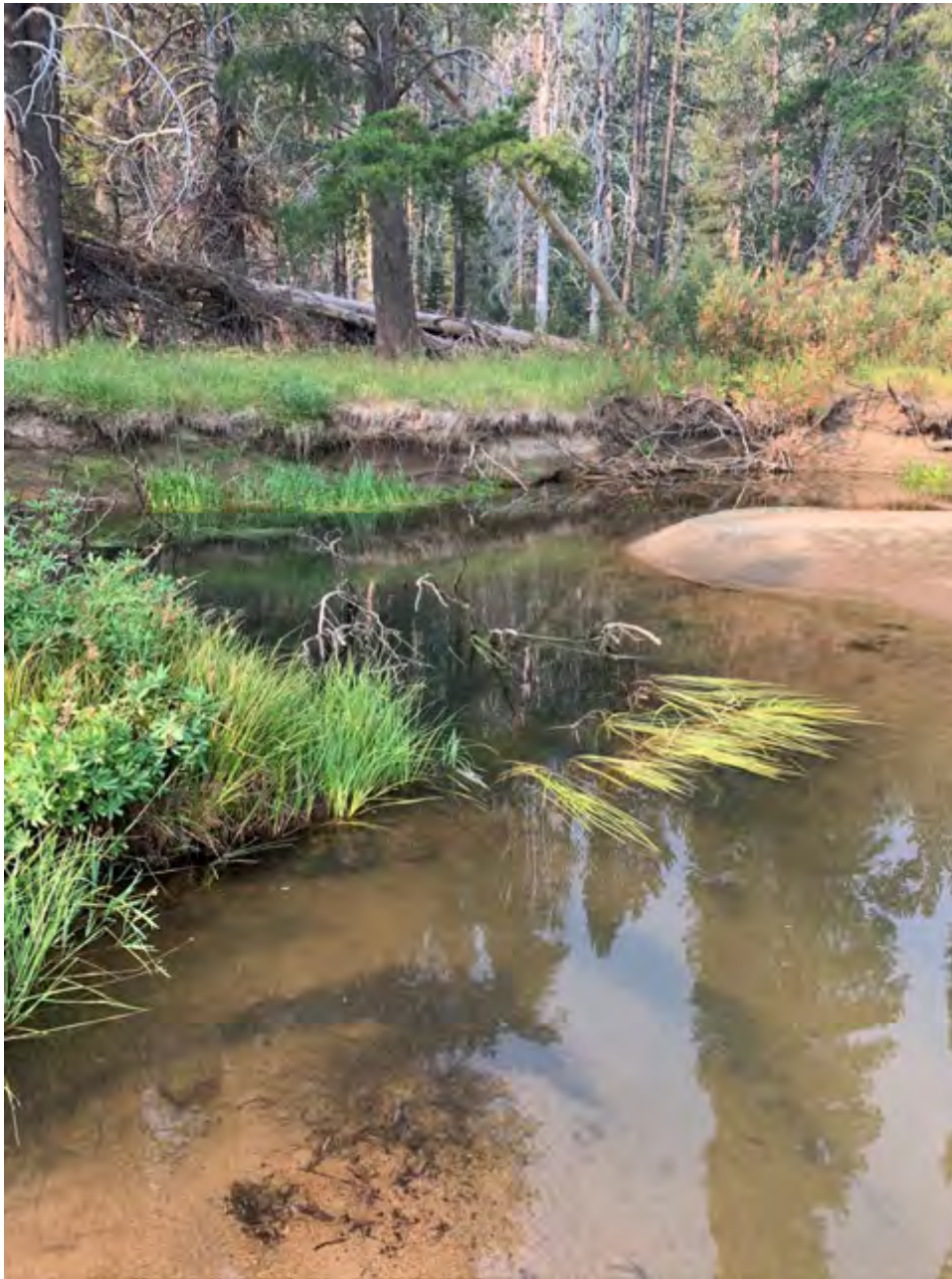
Photo 1. Reach CV-1 showing bank erosion, undercut banks and in-stream woody debris; fine sediment common in this reach.
