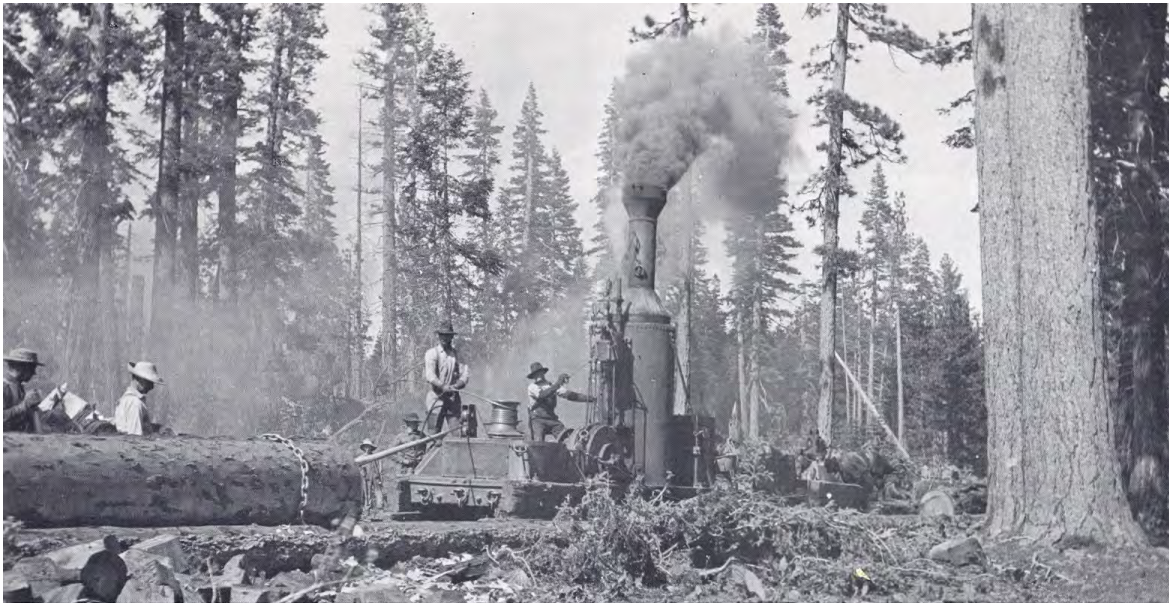
Photo 9. The Dolbeer steam donkey skidded logs through the woods more efficiently than oxen and could hoist logs onto rail cars (courtesy George D. Oliver Collection In Myrick 1962:444)
