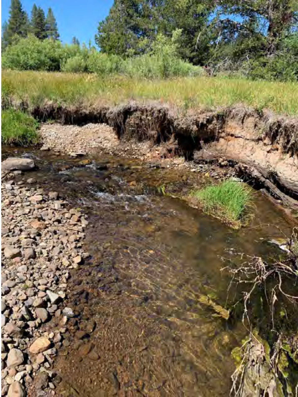
Photo 12. Reach EV-2 showing bank failure and small amounts of in-stream cover; larger (50–100mm) angular cobbles likely coming from Crabtree Canyon tributary, which enters the South Fork near this location.
