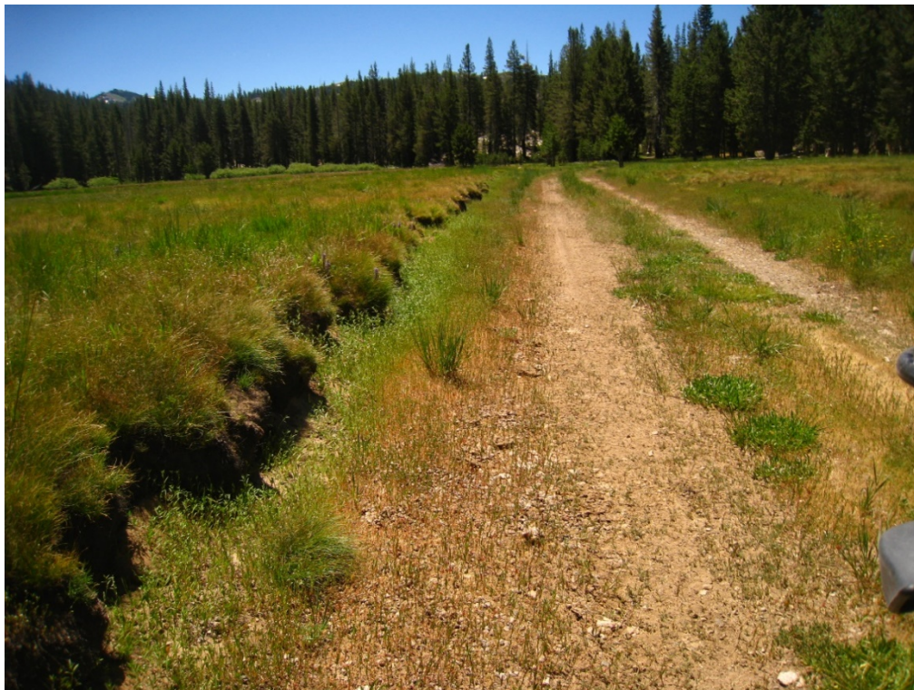
Figure 3-3 Example of Road Runoff Concentrated in a Natural Channel, Upper Lacey Meadow, Reach I (a).
