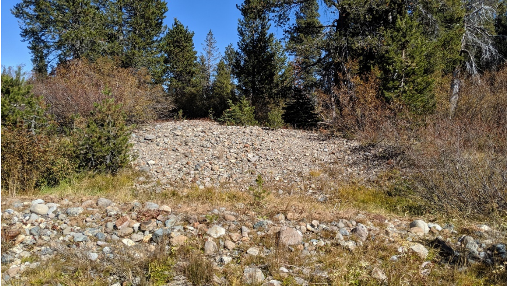
Figure 3-7 Former Channel Blocked by a Push-up Dam in Location Identified in Figure 3-6, Reach H-G Transition. This dam encouraged channel avulsion to the northern side of the meadow and through the forest, depriving meadow of hydrologic support.
