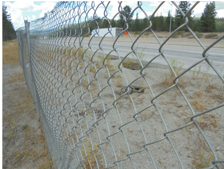
Figure 4. Site 4, existing drainage inlets along freeway near location of proposed swale outlet (low point of freeway/shoulder grade in project vicinity); drainage outlets to remain in place with grass-lined swale as secondary/redundant filtration system; notice erosion from runoff bypassing drainage inlets.
