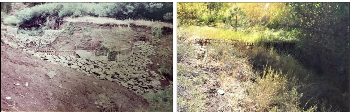
Figure 5. Canyon 4 in 1978 when metal grade control structures were installed (left) and one of those structures in 2019 (right).
