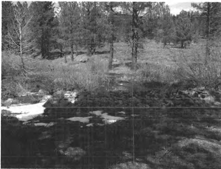
Photo ID# 3, Wing Dam, Segment 1, north of Road 860, view to north. Breach or wash-out in grade can be seen north of the rock alignment where standing water is present.
