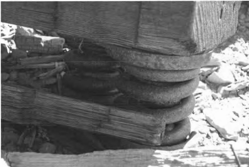
Heavy springs under base of structure.
