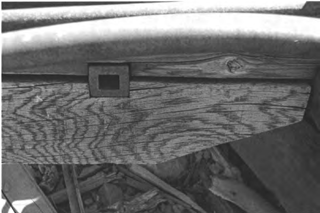
Close-up of wooden skid under base of structure.
