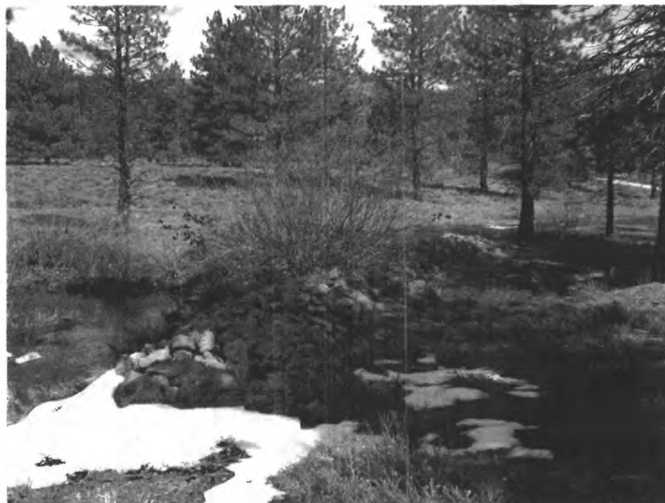
Photo ID# 2, Wing Dam, Segment 1, north of Road 860, view to the east. The creek has breached the grade to the right of the rock alignment.
