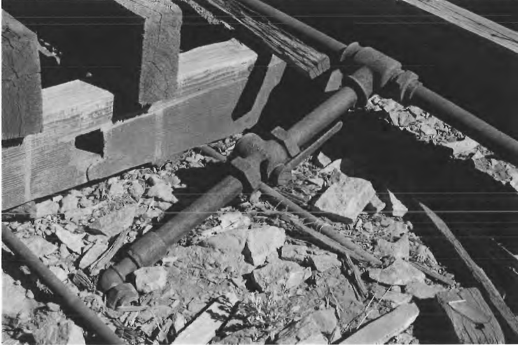
Close-up of water(?) pipe and shut-off valve at center of structure base.
