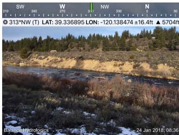
Bank failures could be stabilized to minimize chronic sources of sediment.
