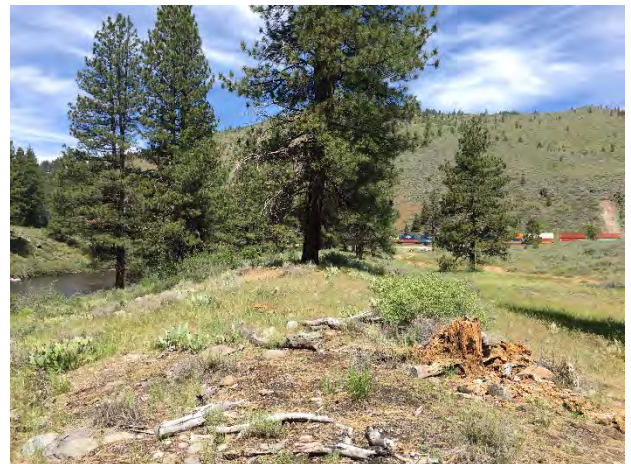
Railroad spur grade channelizes river and limits floodplain inundation
