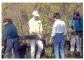
Wattles are installed at the toe (bottom) of the slope, around the OHWM by excavating a trench similar in size to the wattle. Place the wattle in the trench and stake it in place using live stakes through and at the base of the wattle. Bury the wattle, leaving just the top slightly exposed. Excavate additional trenches on the contour of the slope spaced 2' apart as needed, most areas will only need one to two levels of willow wattles. Install wattles in each trench as described above.
