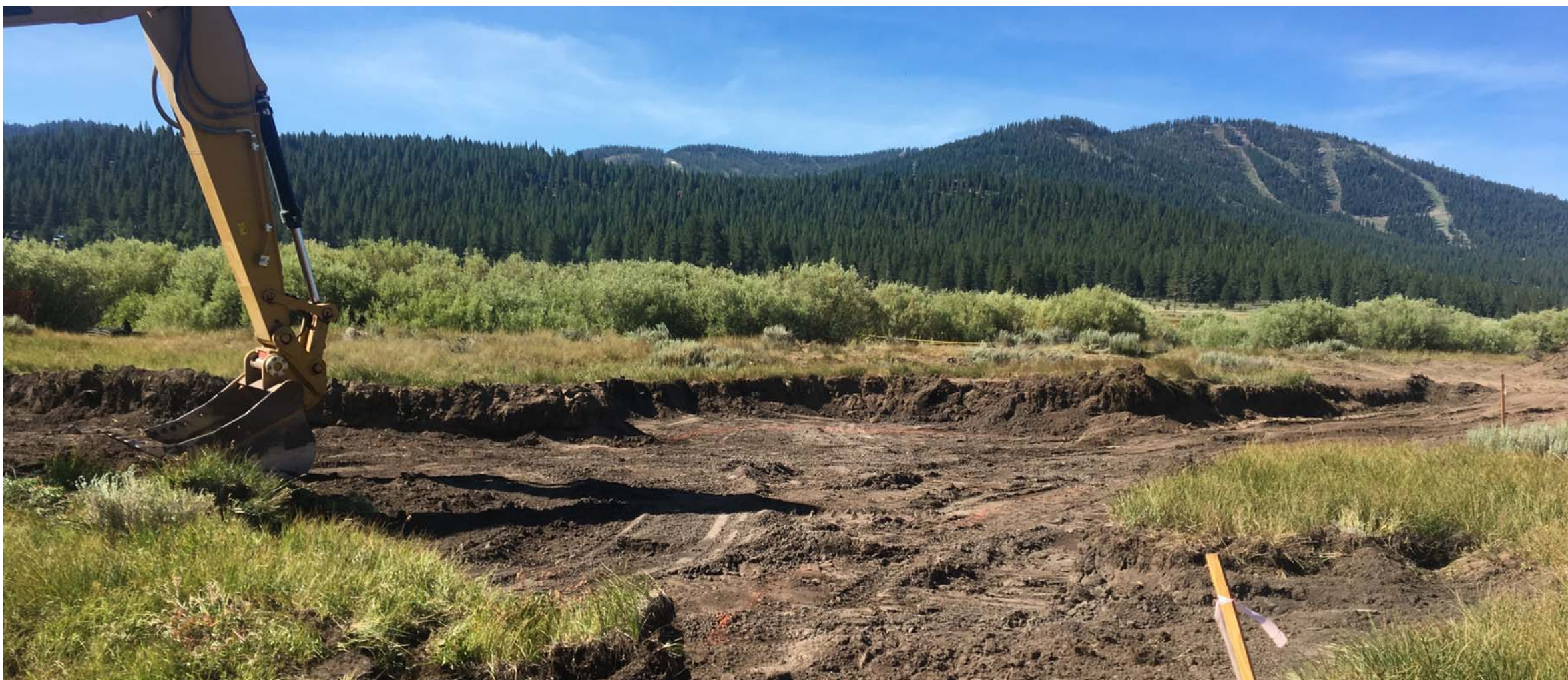
Creating an inset floodplain – salvage and grading
