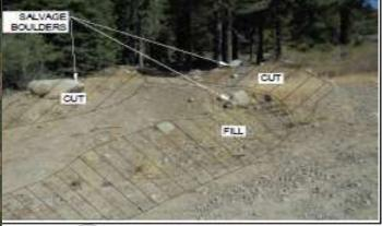
3 SPUR ROAD 3 GRADING DETAIL
