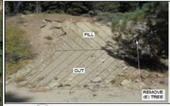
SPUR ROAD 1 GRADING DETAIL
