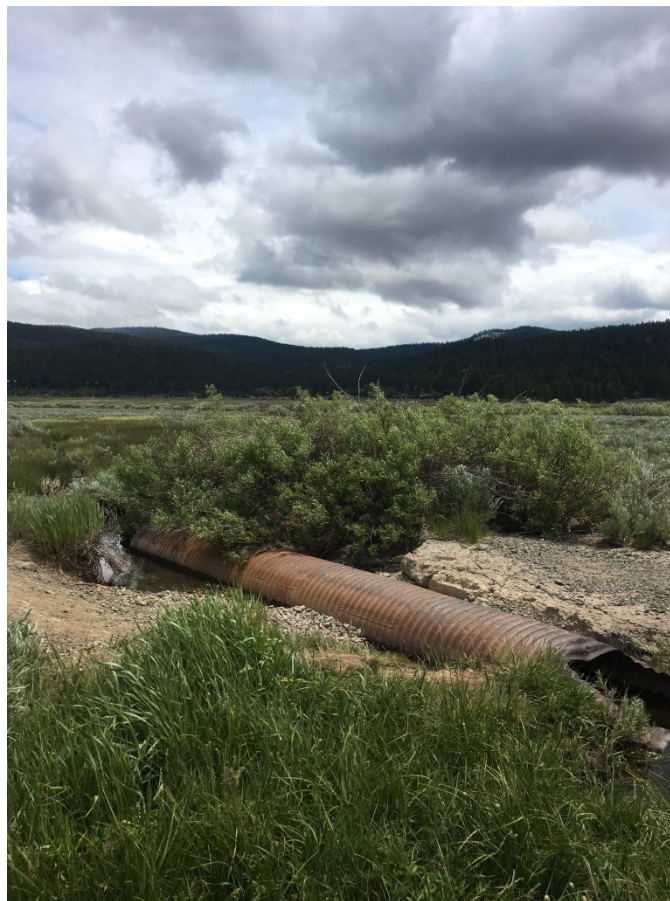
Figure 3- Western culvert on unnamed tributary to Martis Creek. Culvert has been eroded and exposed. High flow events exceed current culvert capacity.
