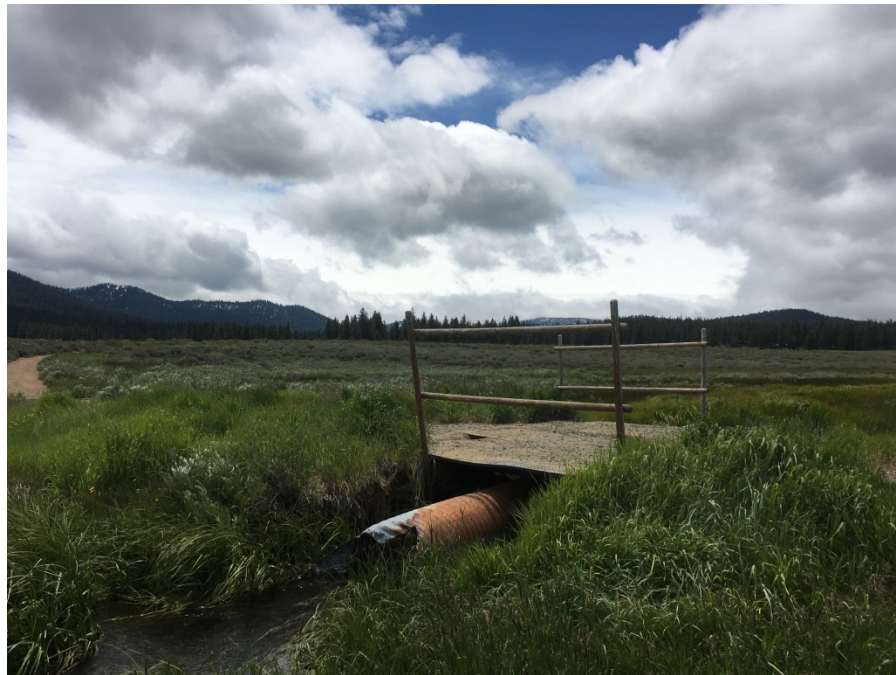
Figure 1- Eastern culvert along unnamed tributary to Martis Creek. Culvert has failed and has eroded under the current recreational trail bridge.
