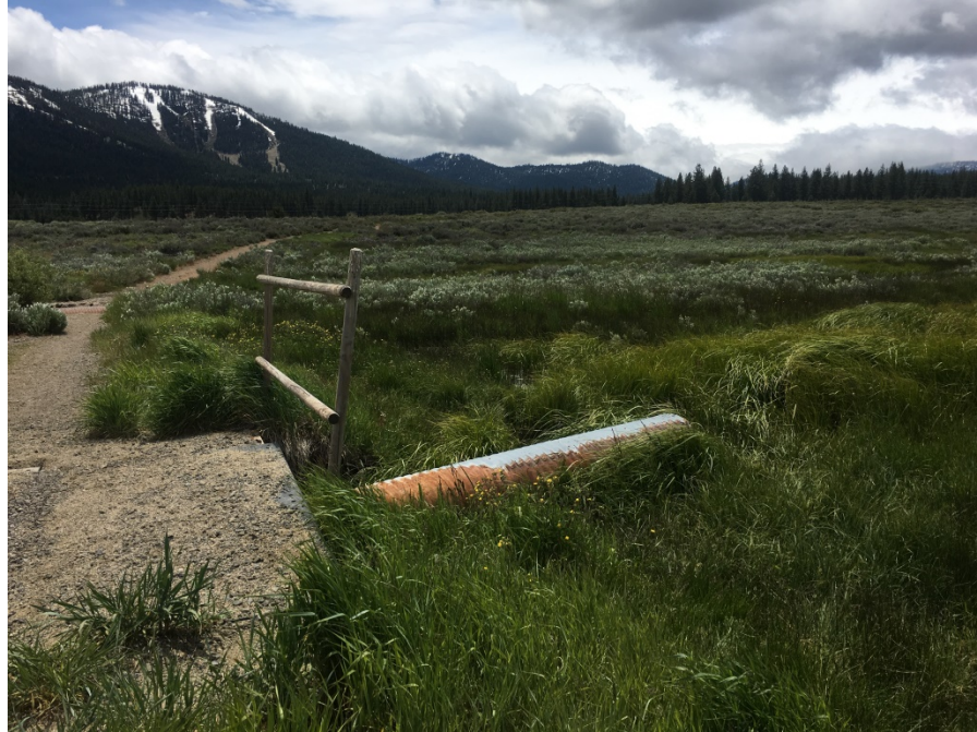
Figure 2- Eastern culvert along unnamed tributary to Martis Creek. Culvert has failed and is breached on north side of recreational trail.
