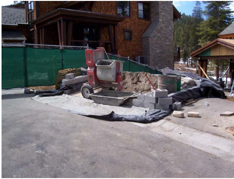
Figure 1: Proper Concrete/Grout Mixing and Containment Station
