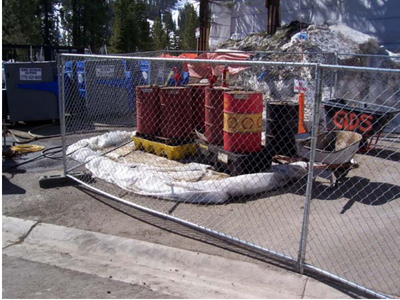
Figure 1: Example of fueling station containment setup.
