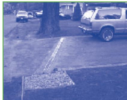
This gravel drain filters pollutants out of driveway runoff.
