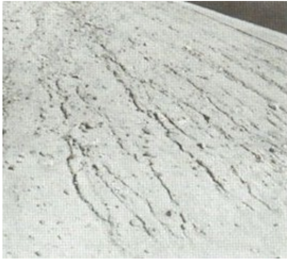
Small channels running down slopes after a heavy rain are evidence of what is called “rill erosion”
