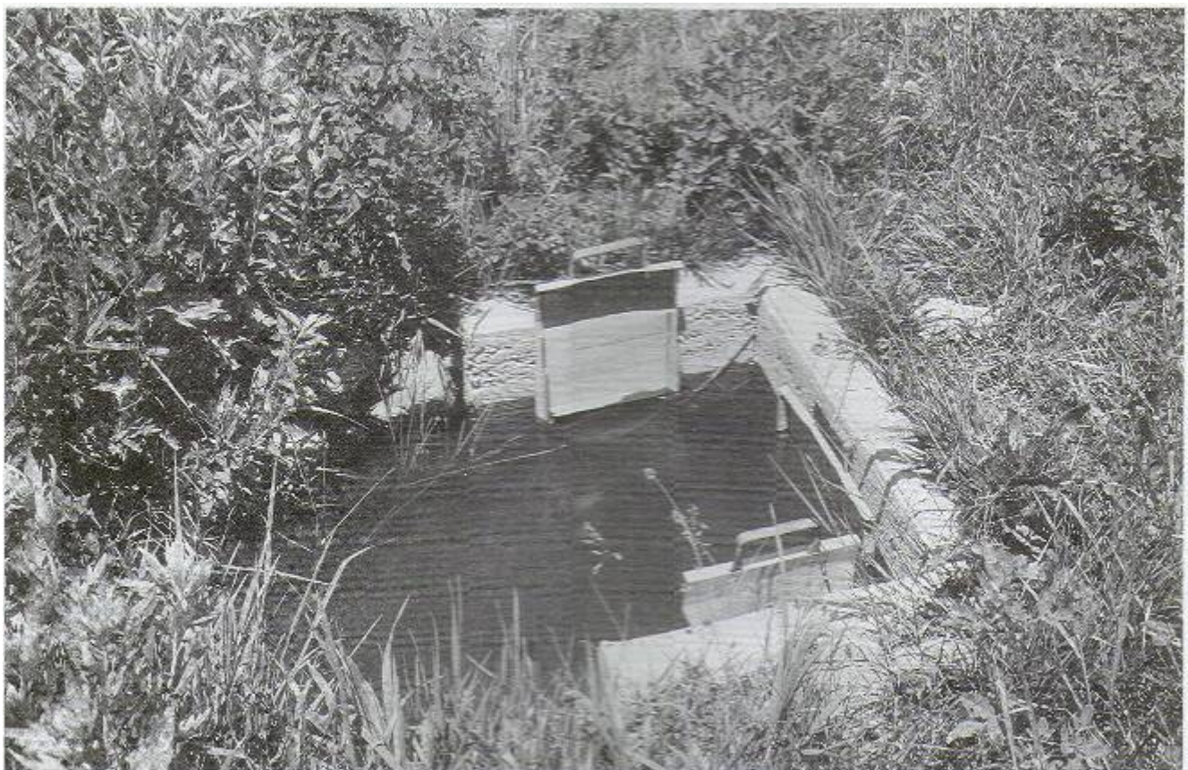
A concrete check structure with slide gates allows control of irrigation flows and minimizes maintenance requirements.
