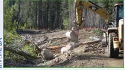
After: The eroding bank in the "before" shot has been re-graded to a sustainable angle and replanted with willows. Note the significant expansion of floodplain area.
