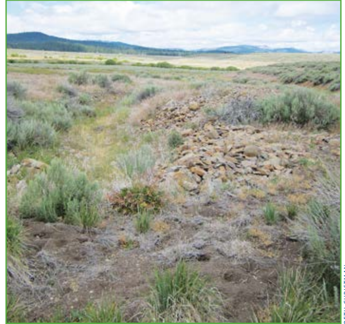
Fill was placed in the channel during reservoir construction, causing downstream erosion. The fill will be removed to prevent future erosion.
