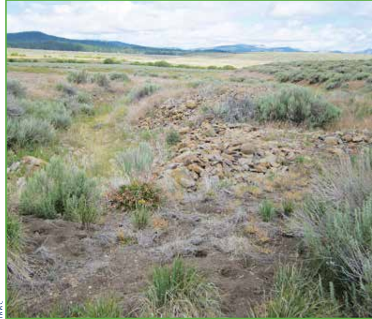
Fill was placed in the channel during reservoir construction, causing downstream erosion. The fill will be removed to prevent future erosion.
