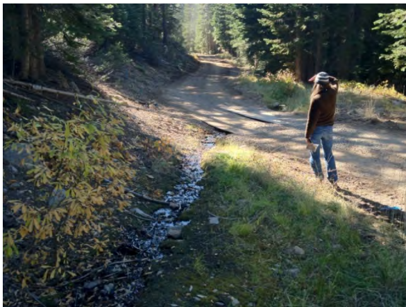
Spring feeding Kiwi Creek. Note use of trench plates to minimize road impacts. (photo credit: Kevin Drake, IERS)
