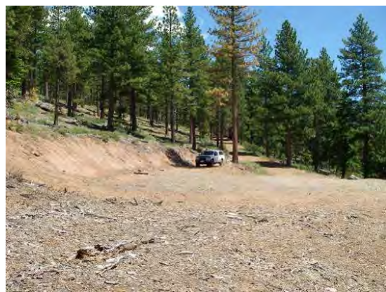
Landing 1 (L1) – large landing with eroding cut and fill slopes. (photo credit: Kevin Drake, IERS)
