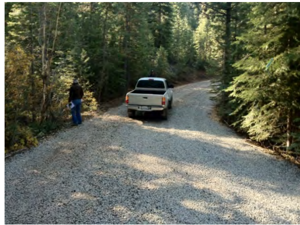
Road armored with rock at small tributary crossing. (photo credit: Kevin Drake, IERS)
