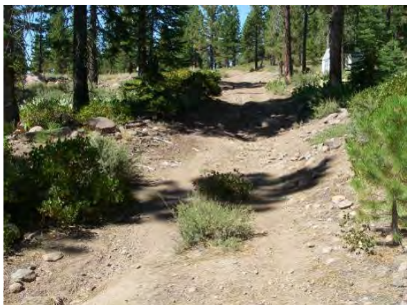
Site P – evidence of erosion and water capture on the main road. (photo credit: Kevin Drake, IERS)
