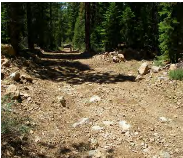
Site B – accelerated erosion on haul road above Dry Lake. (photo credit: Kevin Drake, IERS)
