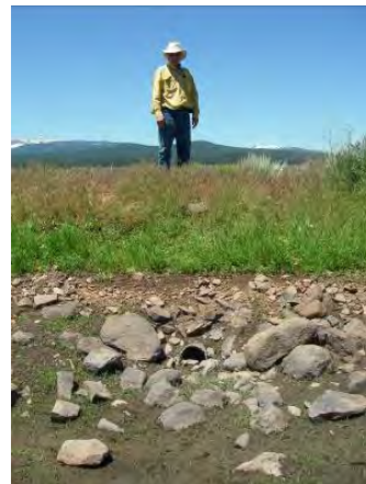
Site I – undersized culverts under road are clogged and insufficient to convey surface water to west side of road impoundment.(photo credit: Kevin Drake, IERS)
