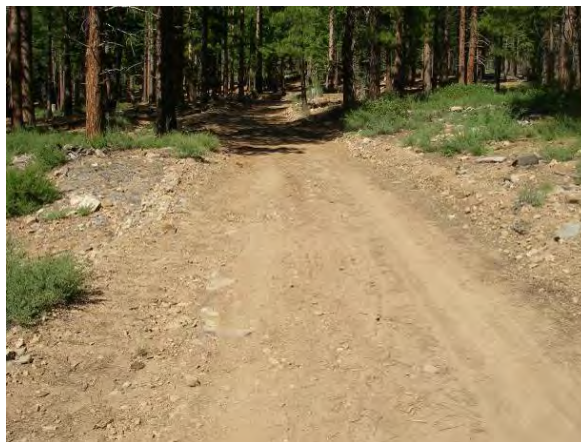
Site E – one season after smooth grading, rilling was observed in the exact same location as the gully. (photo credit: Kevin Drake, IERS)
