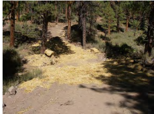
Site F – haul road with unimproved crossing at ephemeral drainage to Martis Creek Lake. Straw was spread after logging in 2009 as a best management practice. (photo credit: Kevin Drake, IERS)
