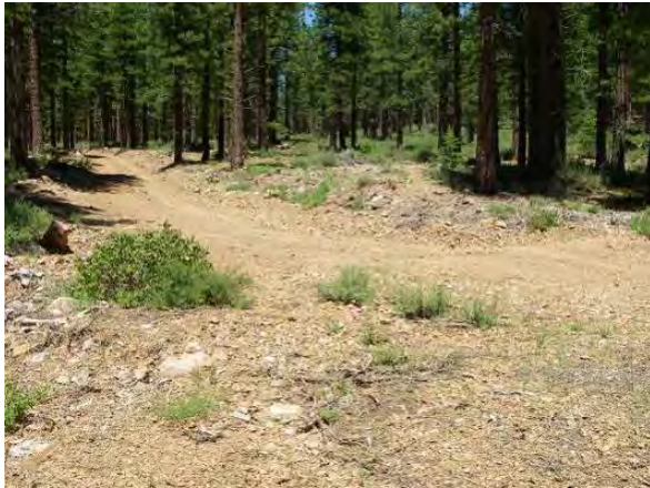
Site C – road runoff connects directly to ephemeral drainage. (photo credit: Kevin Drake, IERS)
