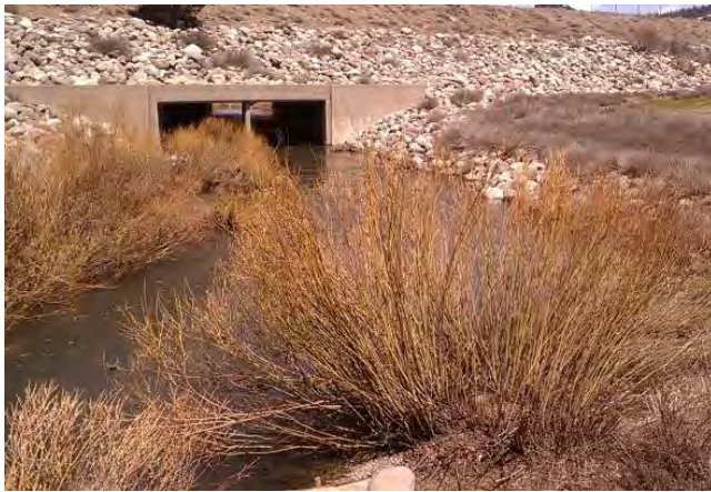
Reach 6 – Martis Creek modified channel at Highway 267. Historical aerial photography indicates that incision episodes correspond with various iterations of highway and channel modification in this location. (photo credit: David Shaw, Balance Hydrologics)
