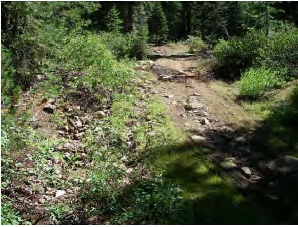
Landing 36 – runoff from this heavily compacted landing drains directly to stream channel (Reach 15). (photo credit: Kevin Drake, IERS)
