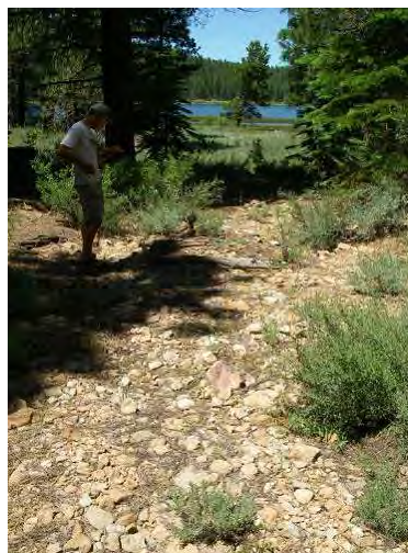
Site A - ephemeral drainage crossing old road above Dry Lake. Headcut has developed just downslope of road. (photo credit: Kevin Drake, IERS)
