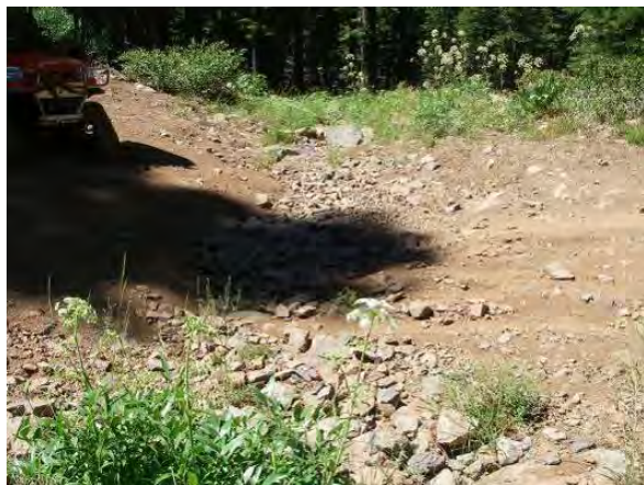
Site S – crossing is fairly stable but could benefit from broadening and armoring sideslopes. (photo credit: Kevin Drake, IERS)
