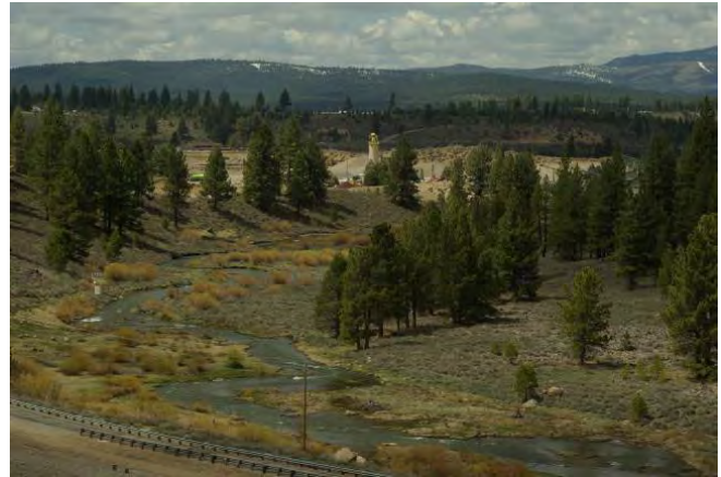
Reach 11 – Grade-controlled channel and meadow downstream of Martis Dam. Streamflow in this photograph is approximately 180 cfs, slightly lower than the estimated 2-yr flow. (photo credit: Brian Hastings, Balance Hydrologics)
