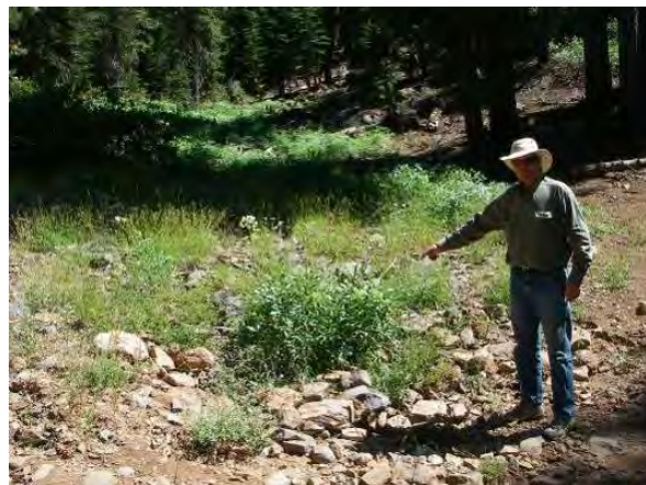
Site S – hand-placed rock above road for energy dissipation and sediment capture in ephemeral drainage. (photo credit: Kevin Drake, IERS)
