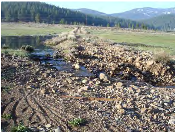
Site I – road impoundment interrupts meadow flooding patterns, causing intermittent road damage and vehicle access issues. (photo credit: Kevin Drake, IERS)
