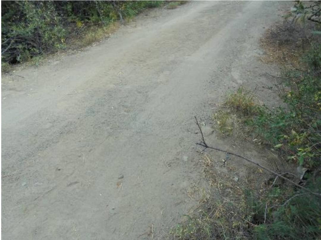
Photo 18. #3 – Quarry culvert outlet from basin (looking south).
