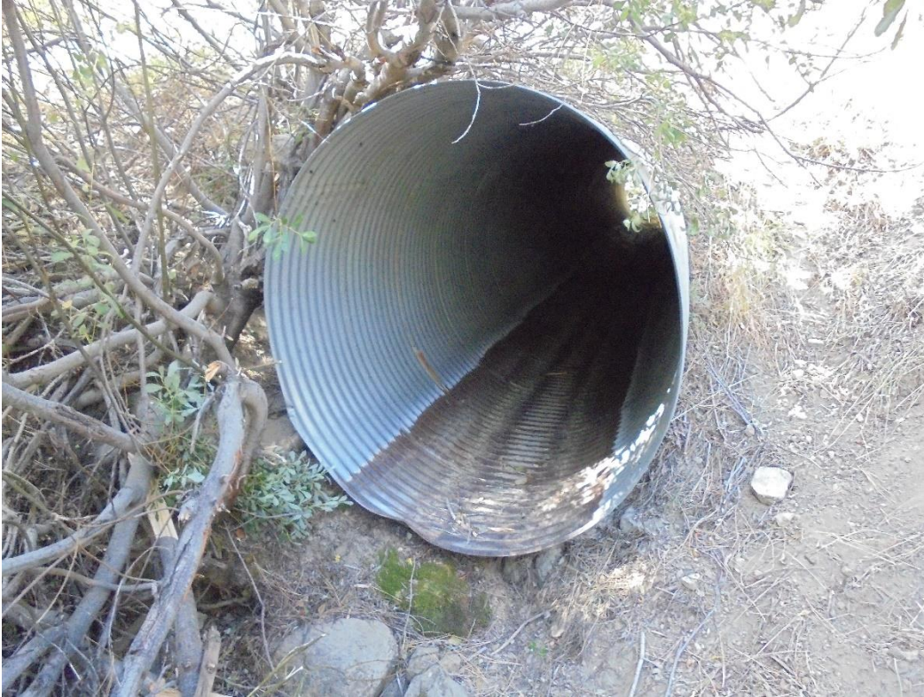
Photo 41. #10 – Crossing #4 culvert outlet (looking northwest).
