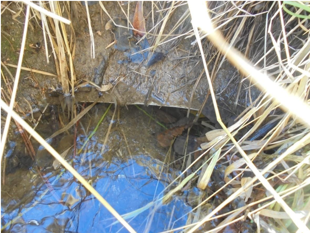
Photo 36. #8 – Crossing #3 culvert outlet approximately 80% full of sediment.
