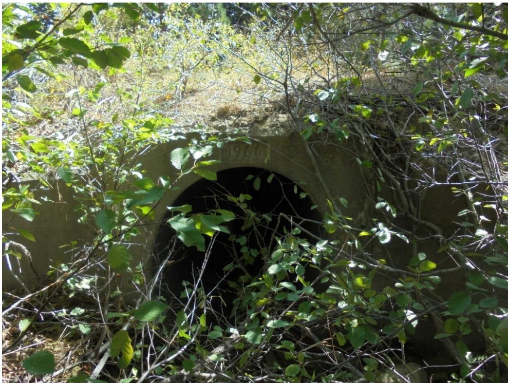
Photo 40. #10 – Crossing #4 culvert inlet (looking south).
