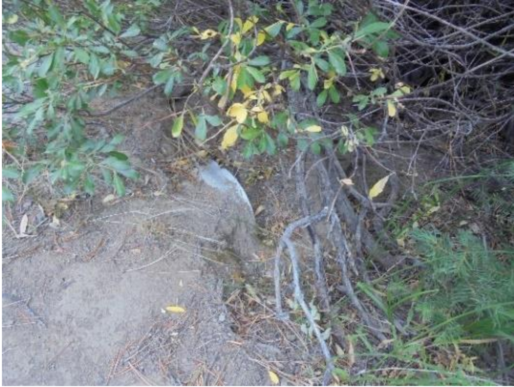
Photo 19. #3 – Quarry culvert inlet (looking southwest).
