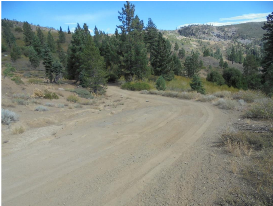
Photo 3. Gullying along northern edge of #1a – Billy Mack Road Ascent to Ridge (looking northeast down road from start of #1f – OHV South Loop).
