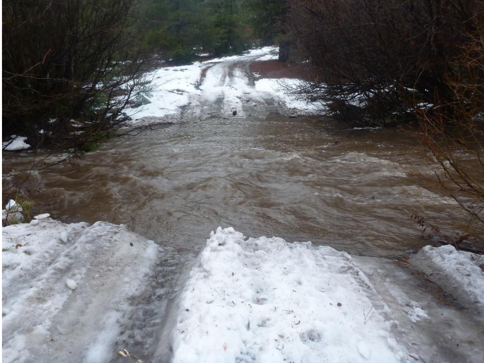
Photo 89. #14 – Crossing #5 Gregory Creek east fork flowing over Billy Mack Road due to high flows during storm in fall 2016 (looking northwest, up Billy Mack Road).
