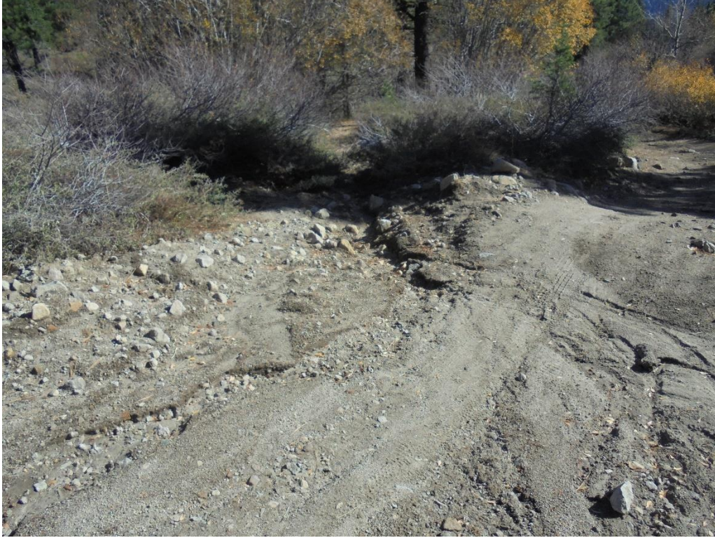
Photo 69. Example of erosive rilling and gullying from inadequate waterbar spacing on Billy Mack Road (taken in November 2016 after large October 2016 storms).
