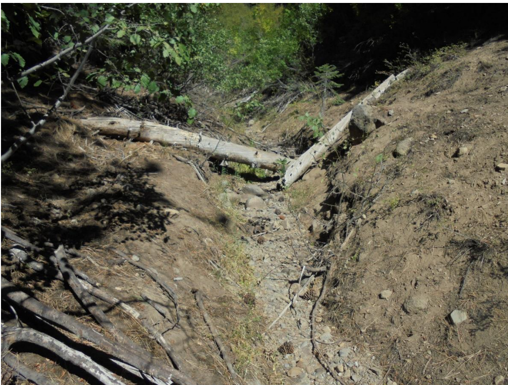
Photo 42. #10 – Crossing #4 immediately downstream of culvert (looking south).
