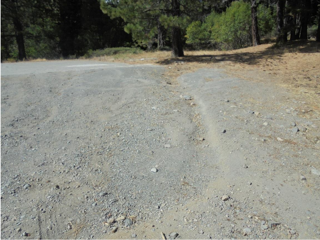
Photo 81. Eroded flowline from northeast corner of #15c – Concrete Pad (looking northwest).
