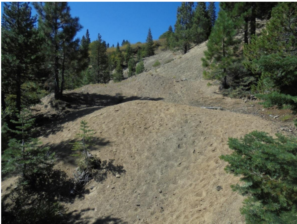
Photo 16. #3 – Quarry north side (looking west from Billy Mack Road).
