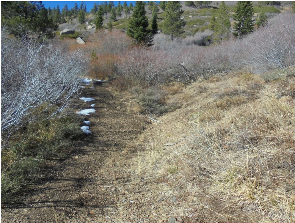
Photo 28. #7 – Project Area C Spur Road capturing drainage causing minor erosion (looking northwest).
