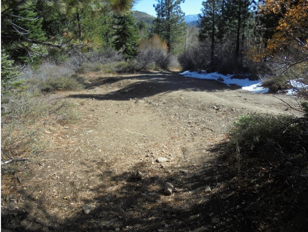
Photo 27. Looking southeast from #6 – Billy Mack Road/DLRT Connector toward Billy Mack Road, waterbar diverts runoff to the left where minor erosion is evident.
