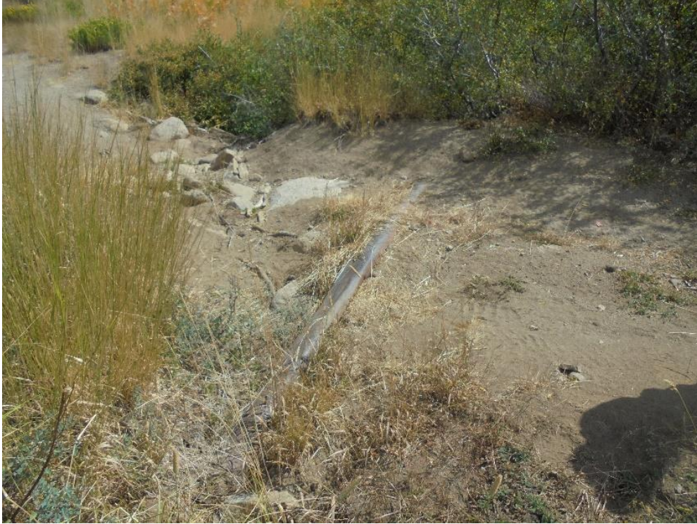
Photo 13. #2 – Southwest Fork USFS Rd 6-inch iron culvert at Crossing #1 (looking southeast in downstream direction).
