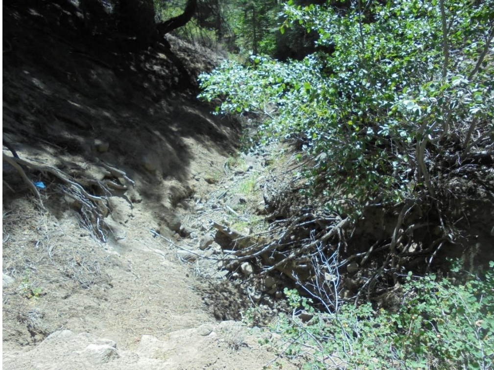
Photo 43. #10 – Crossing #4 approximately 75 feet downstream of culvert outlet (looking south).
