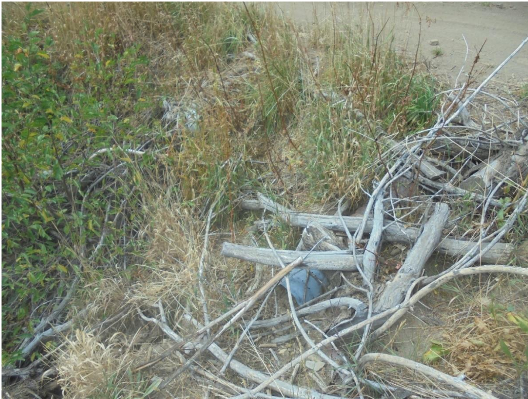
Photo 22. #5 – Crossing #2 culvert outlets (looking west).
