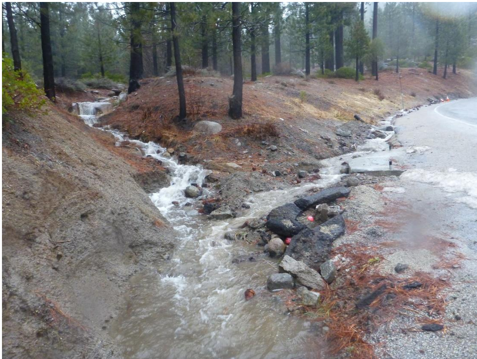
Photo 94. #15 – Confluence of runoff from I-80 West Exit 180 off-ramp and ephemeral drainage from the lower eastern portion of Johnson Canyon (looking north); these flows drain through the Caltrans drainage ditch and join runoff flows from the Former Staging Area before entering Gregory Creek.
