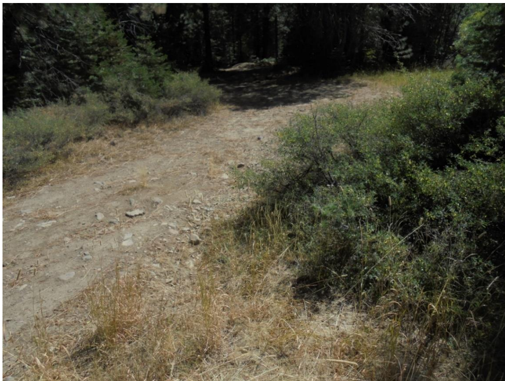
Photo 71. #13 Gregory Creek Spur Road terminus at Gregory Creek overflow channel (looking southeast).
