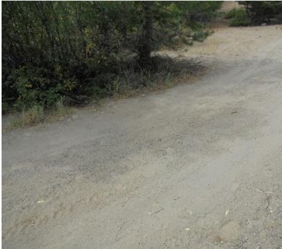
Photo 20. #3 – Quarry culvert outlet area (looking southeast).
