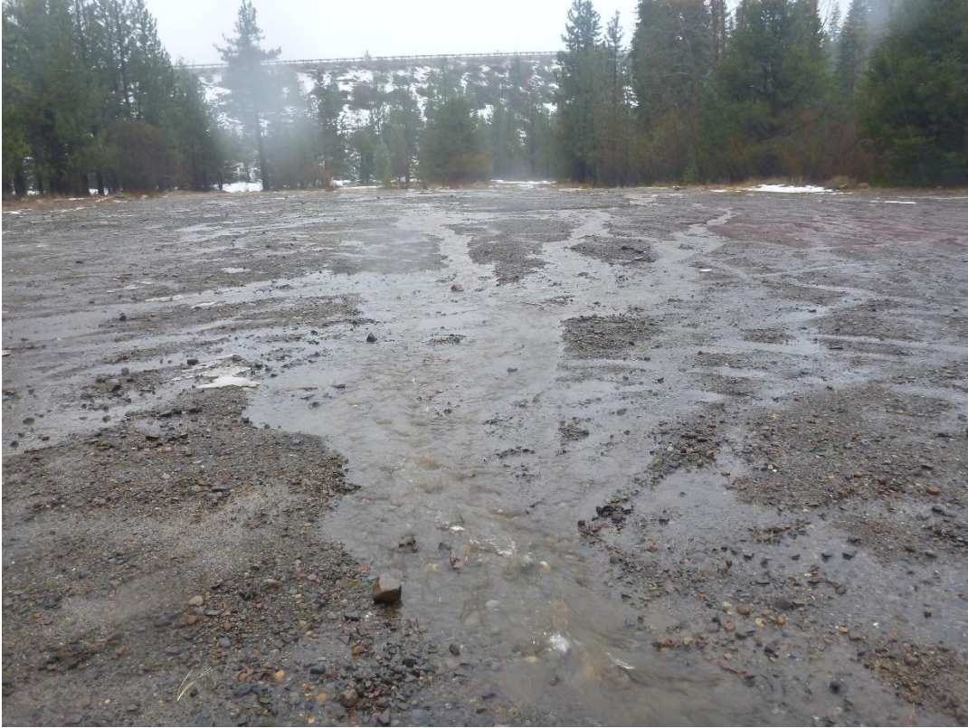
Photo 91. #15d – Compacted Subbase during storm in fall 2016 (looking southwest).
