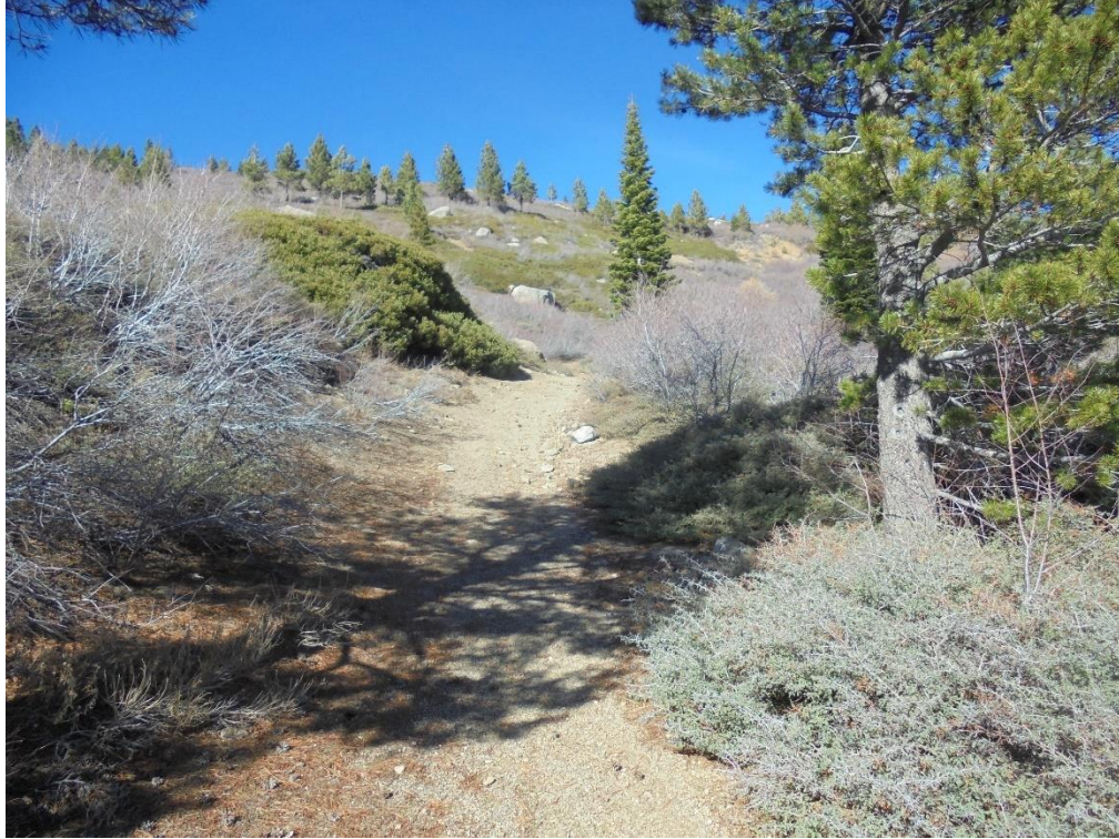
Photo 29. #7 – Project Area C Spur Road capturing drainage causing minor erosion (looking northeast).
