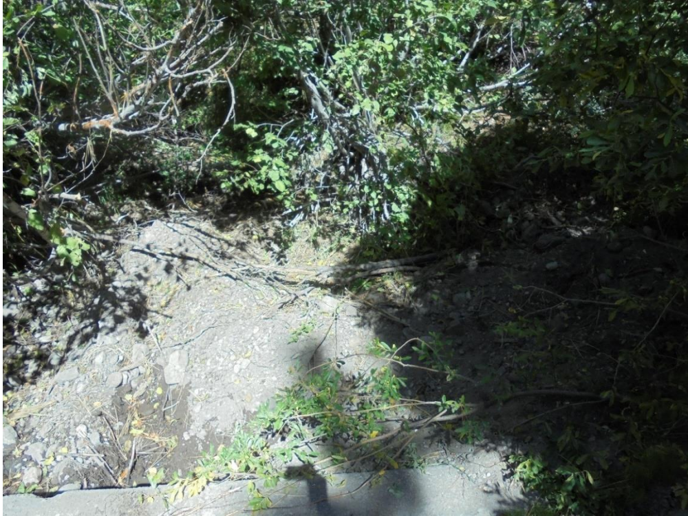
Photo 73. #14 – Crossing #5 Gregory Creek east fork (looking north upstream from Billy Mack Road; lose dirt in channel, possibly from road maintenance crew).
