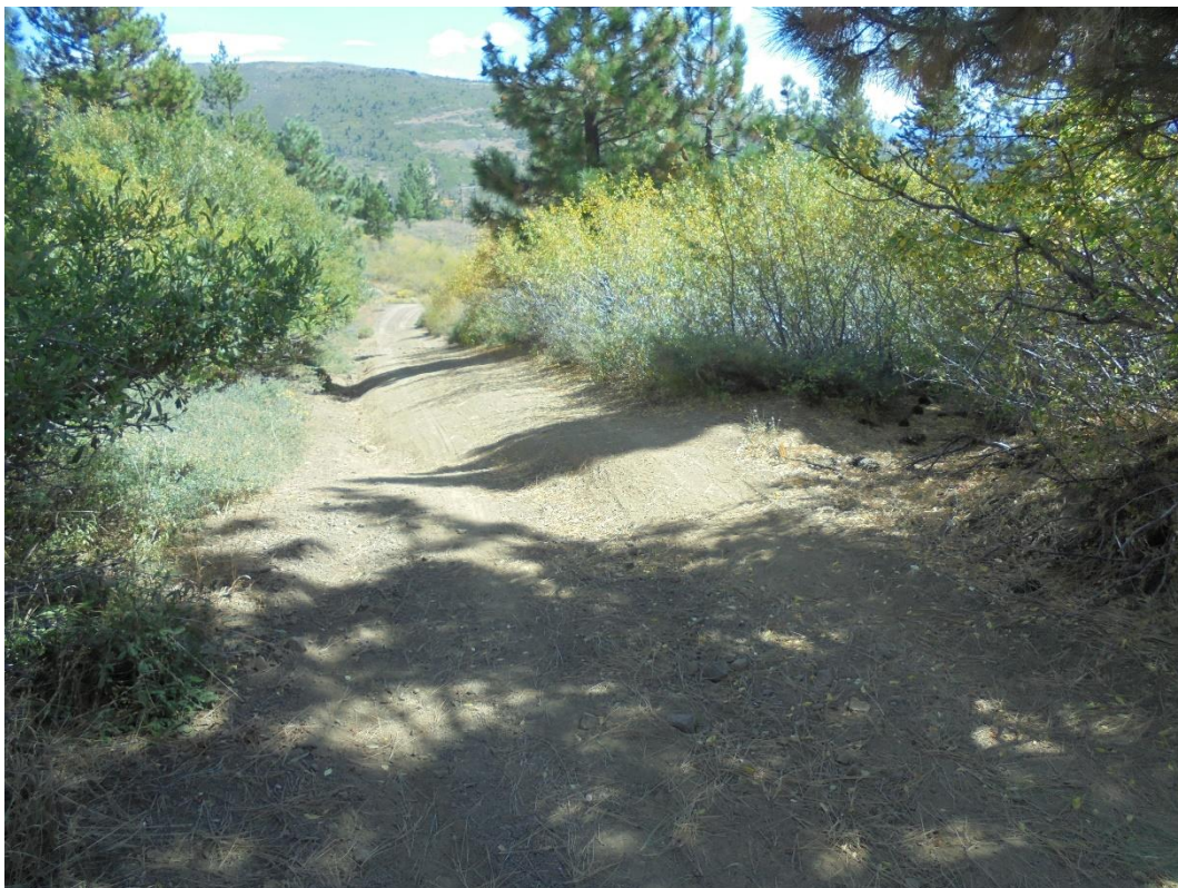
Photo 12. #1g – Rolling Dip at bottom of Four Corners drainage area (looking east from location where OHV Center/North Route fork from Billy Mack Road).
