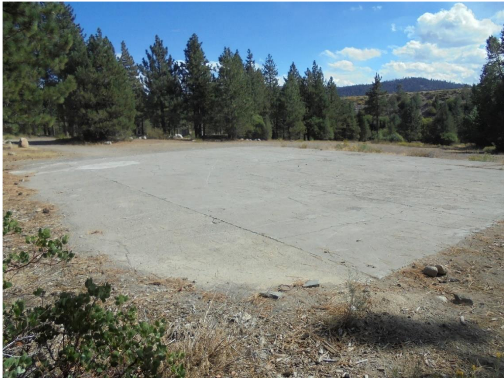
Photo 80. #15c – Concrete Pad covering northwest portion of #15 Former Staging Area (looking southeast).
