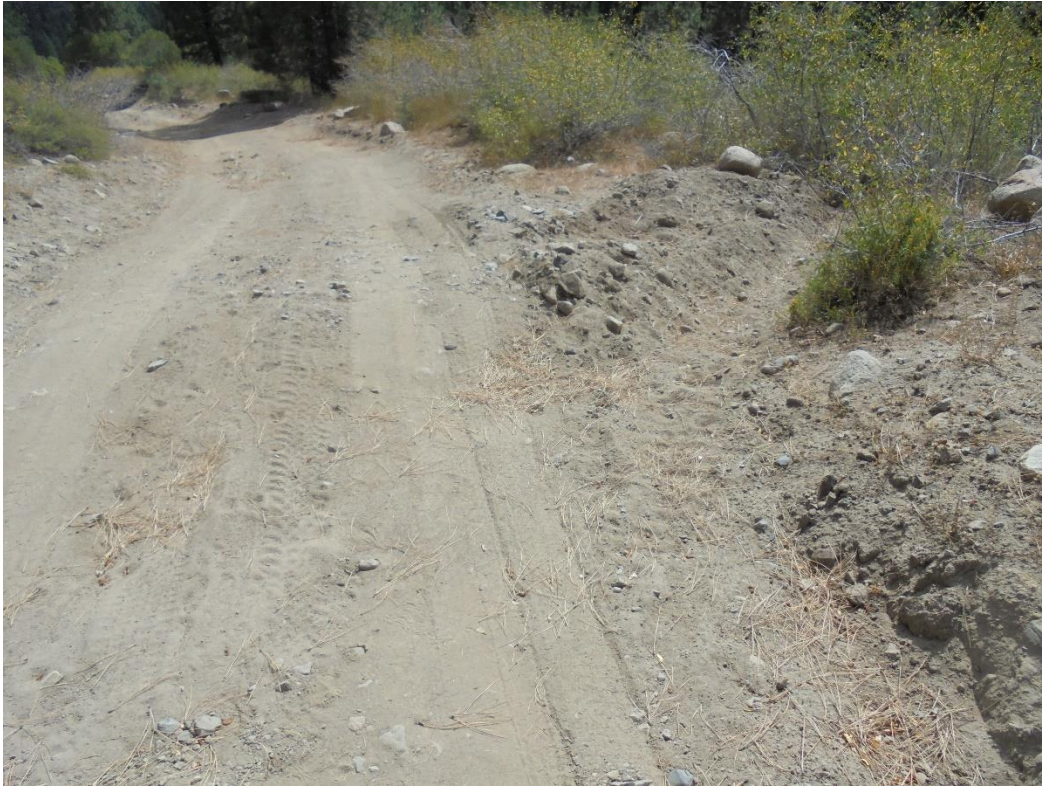
Photo 57. #12 – Billy Mack Road waterbar #1 (from The “T” working down).
