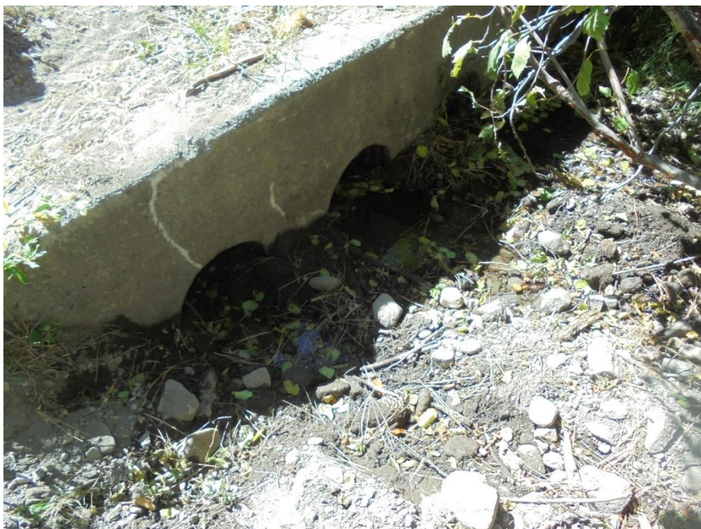
Photo 72. #14 – Crossing #5 Gregory Creek east fork culvert inlet (looking southwest).
