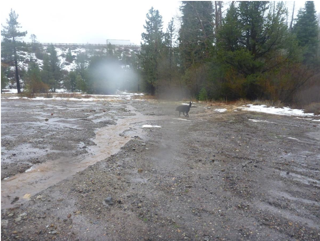
Photo 92. #15d – Compacted Subbase during storm in fall 2016 (looking southwest).
