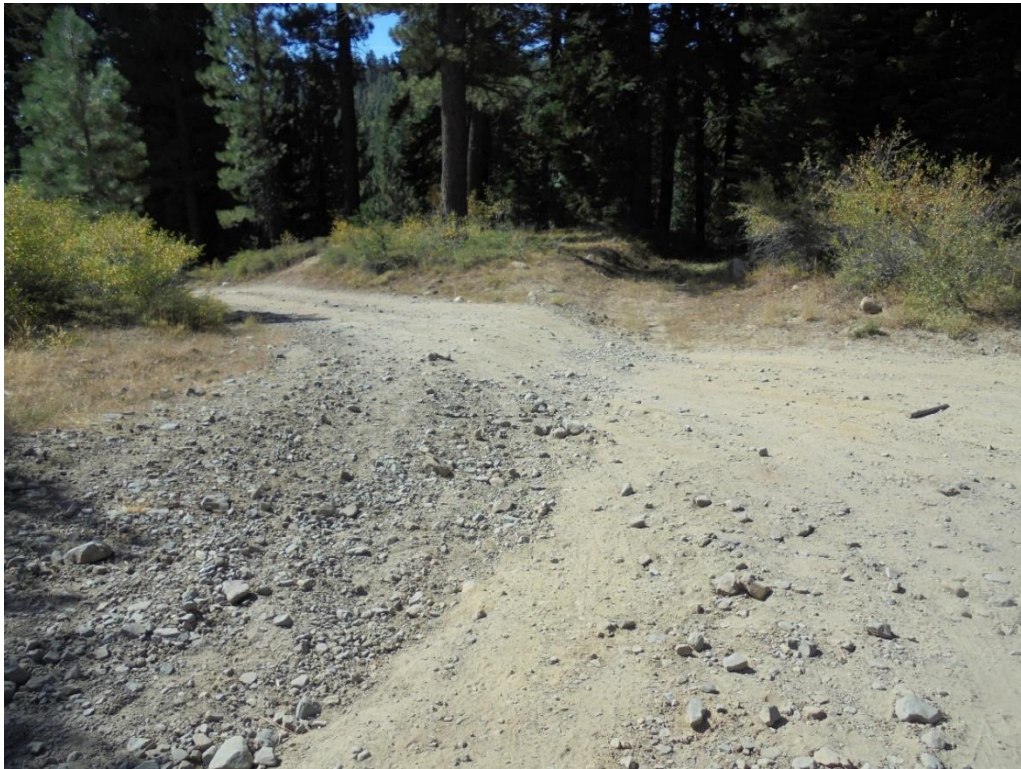
Photo 56. #11f – Billy Mack Road Fork Rolling Dip and Diversion Channel (looking southwest from USFS Road 0676-088 fork).
