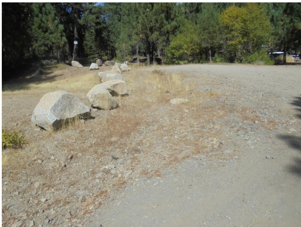
Photo 84. #15e East Drainage along #15 Former Staging Area (looking north upstream from Staging Area access road).
