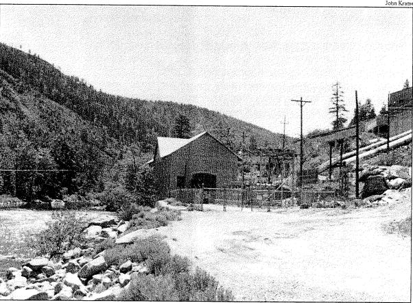
One of Sierra Pacific Power Company's turn-of-the-century hydroplants located in the Truckee River canyon upstream of Reno. Water is brought into the plant by the penstocks on the right edge of the photo.
