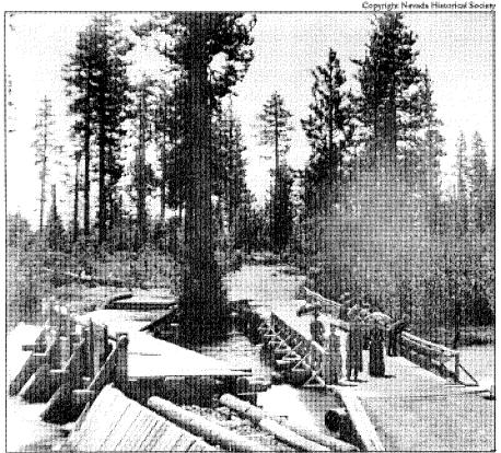
Pedestrians strolling by Von Schmidt's timber crib dam at Lake Tahoe, circa 1880. Note the plank facing showing at the lower left corner.
