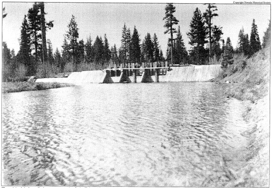
The original timber crib dam constructed at Lake Tahoe. Note the individual planks used for the facing.
