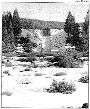
Floodflows at Martis Creek Reservoir are released through this spillway.
