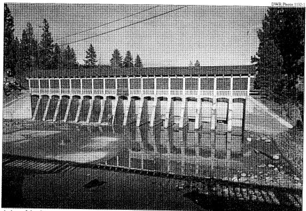
A view of the downstream side of Lake Tahoe Dam under low water conditions. Note the 17 individual gates that regulate releases.
