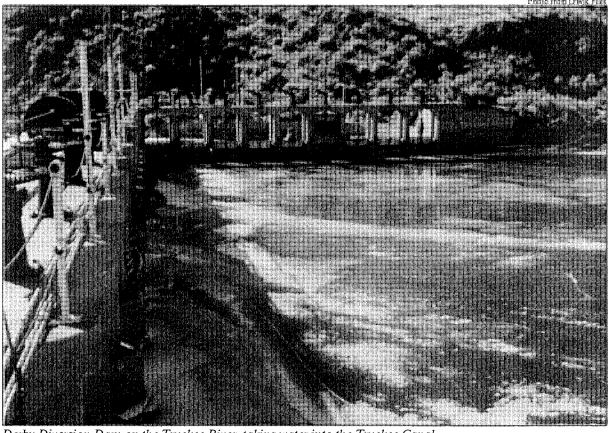
Derby Diversion Dam on the Truckee River, taking water into the Truckee Canal.
