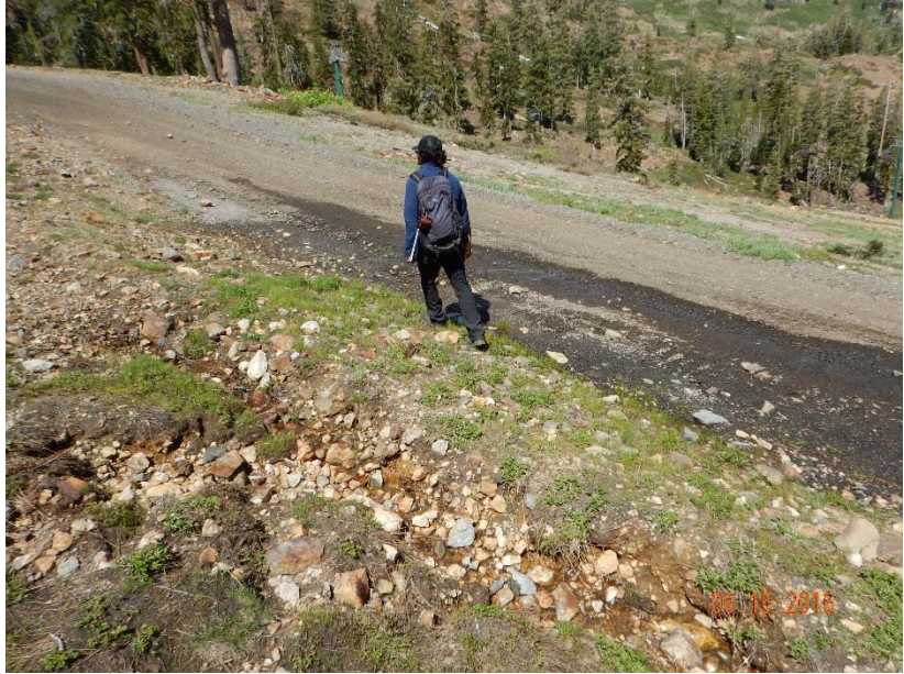
Figure 13. Small channel/ditch forming parallel to road. Water maybe permeating through small berm between road and channel.
