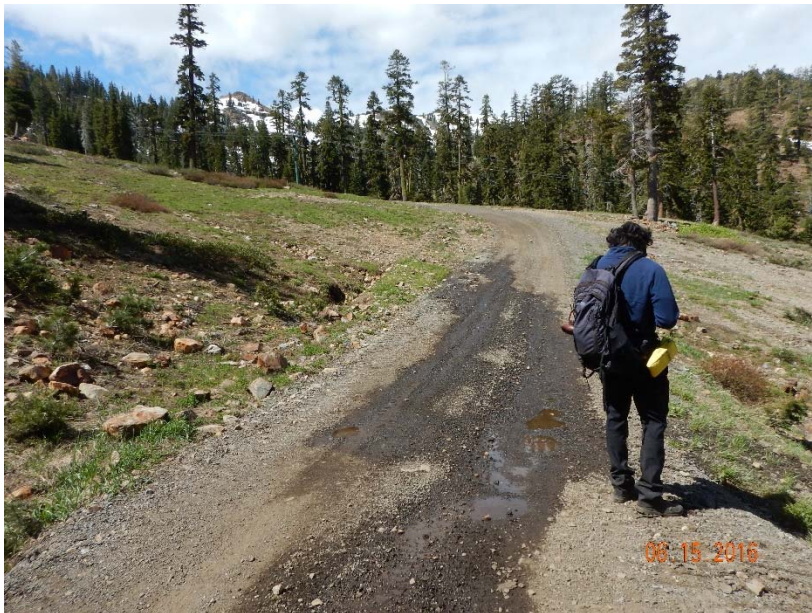
Figure 14. Extent of runoff from small channel/ditch onto road. Runoff travels ~20ft on road.
