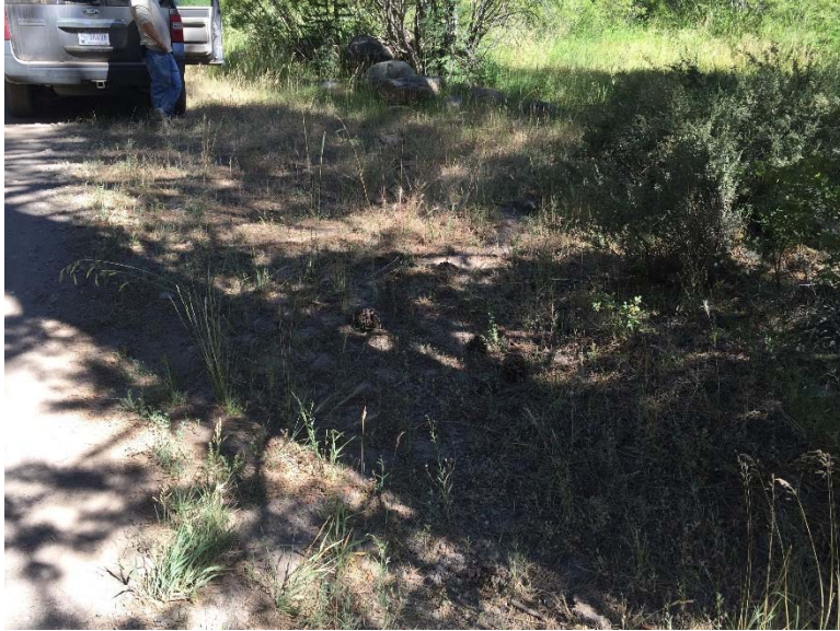
J15: Pullout/landing that captures some runoff and sediment from J6. This area outslopes runoff and sediment into Jackass Creek.
