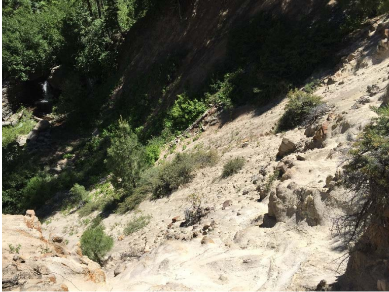
2.11: Segment of road built on toe of a landslide. A washout event may have allowed mass failure of the fillslope. Mass amounts of fillslope is no longer present and has left the remaining fillslope with low vegetation and bare soils.
