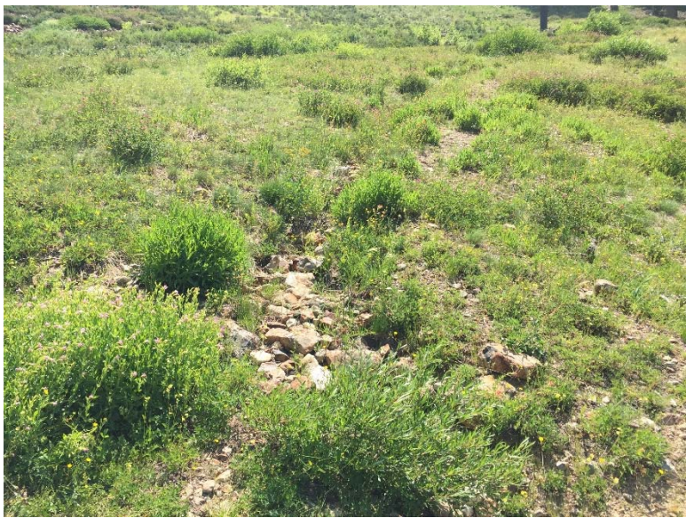
Figure 7. Diverted road surface runoff has created a channel that goes downslope to a lower portion of this switchback.
