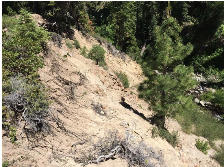
2.12: Exposed cutslope allowing for mass movement of sediment.
