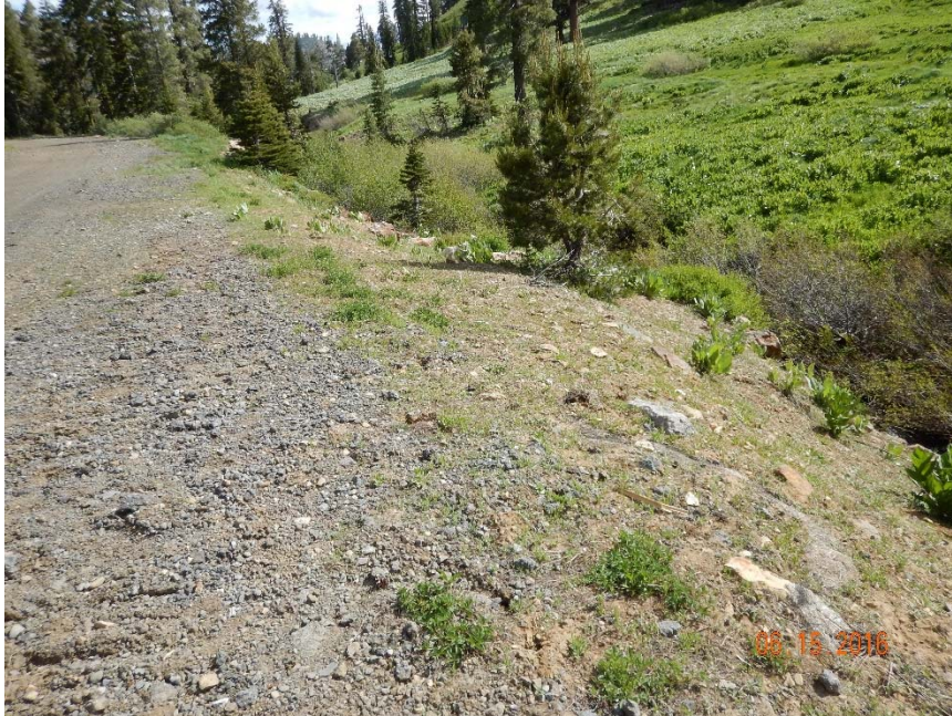
Figure 4. Fillslope of road placed directly into channel.
