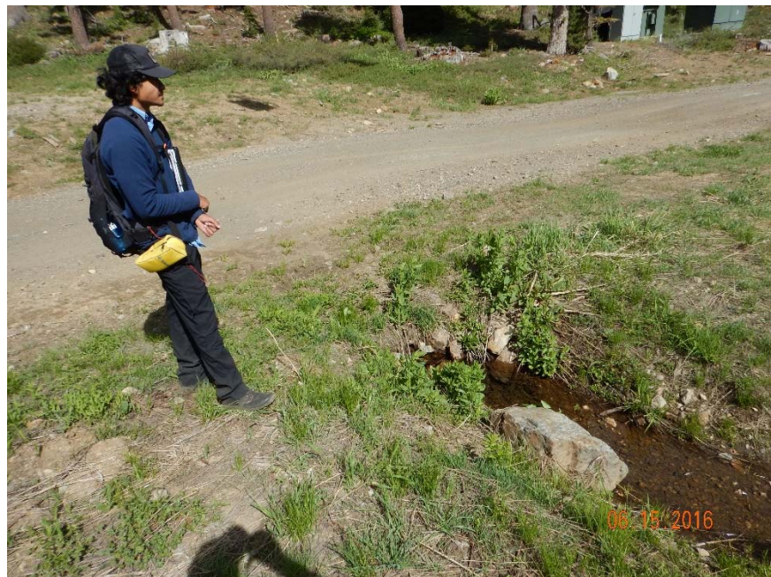
Figure 5. Damaged culvert outlet.
