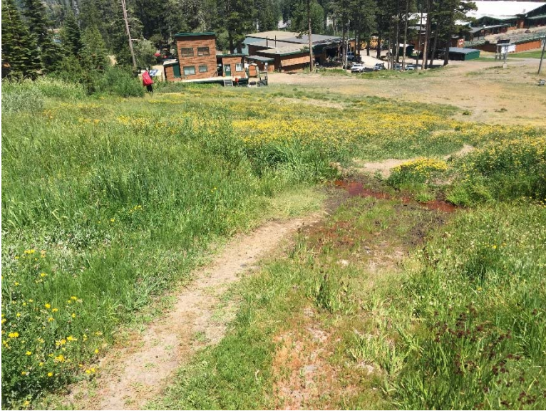
Figure 2. Rillings that have formed from large amounts of surface runoff that have bypassed waterbars.
