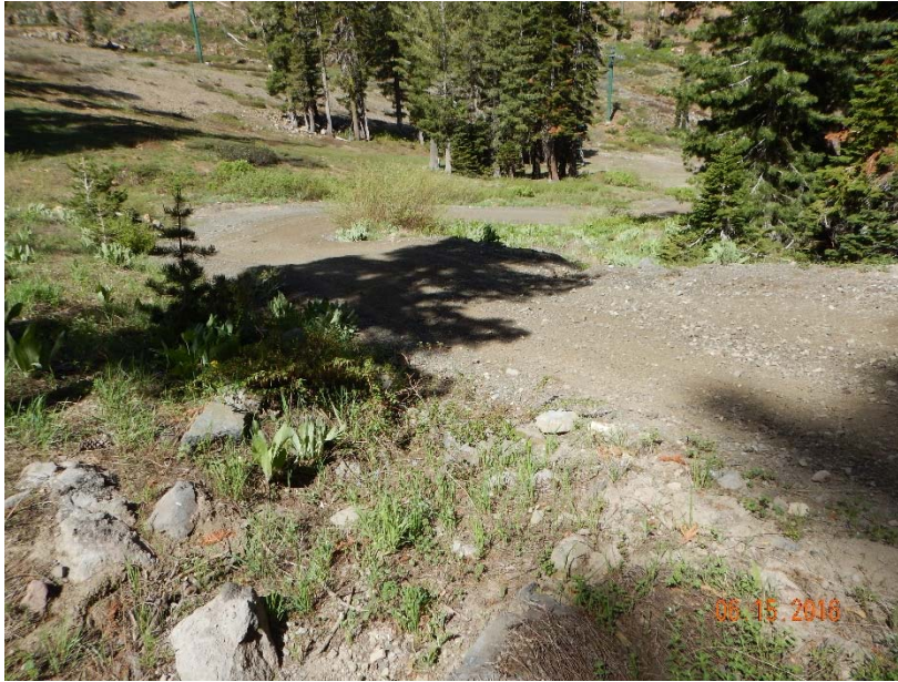
Figure 11. Ephemeral channel crossing road through trough of rolling dip.
