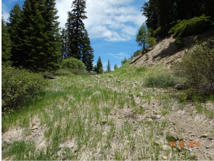
Figure 5. Looking upslope (northeast) at the base of feature C2. Rilling can be seen at center of the photo and moving to the bottom right. Cutslope has exposed surface.
