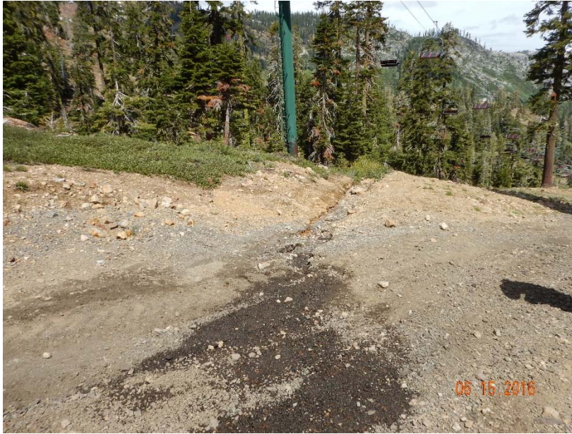
Figure 17. Rilling creating inside ditch on outslope road. Rolling dip transporting larger than normal runoff off road. Outlet is being scoured and incised due to large amount of flow.
