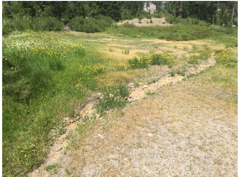
Figure 2. Rillings that have formed from large amounts of surface runoff that have bypassed waterbars.
