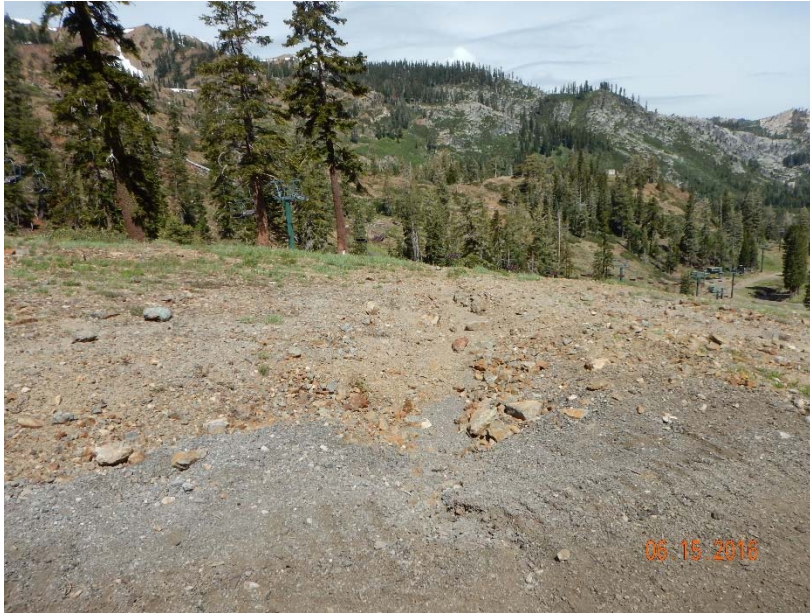
Figure 15. Rolling dip/waterbar transporting large amounts of runoff off the road. Outlet is filled with road material and sediment, and is flowing past the outlet, downslope, towards stream.
