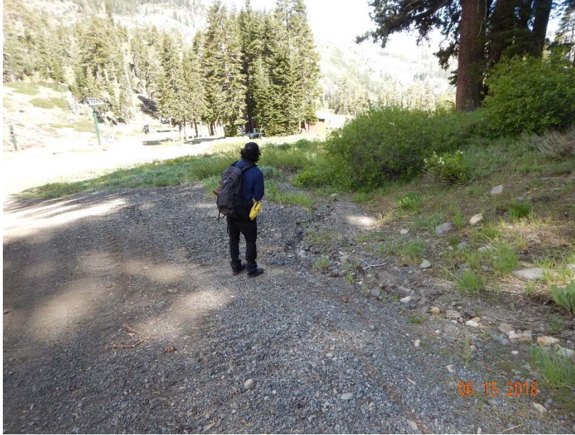
Figure 9. Inside ditch of inslope road shows scouring and rilling. Rilling continues past leadout.
