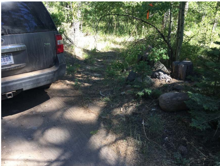
J1. Leadout filled with sediment heading towards channel.
