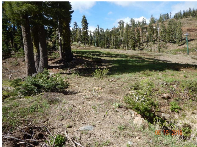
Figure 12. Old road passing over culvert crossing. Runoff from old road flows over top of the culvert outlet and into the stream.
