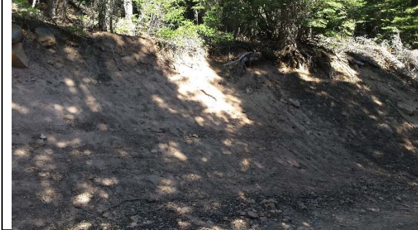
Photo 7a Heading: 270 Massive cutslope is actively eroding. Vegetation is sparsely holding on at top
