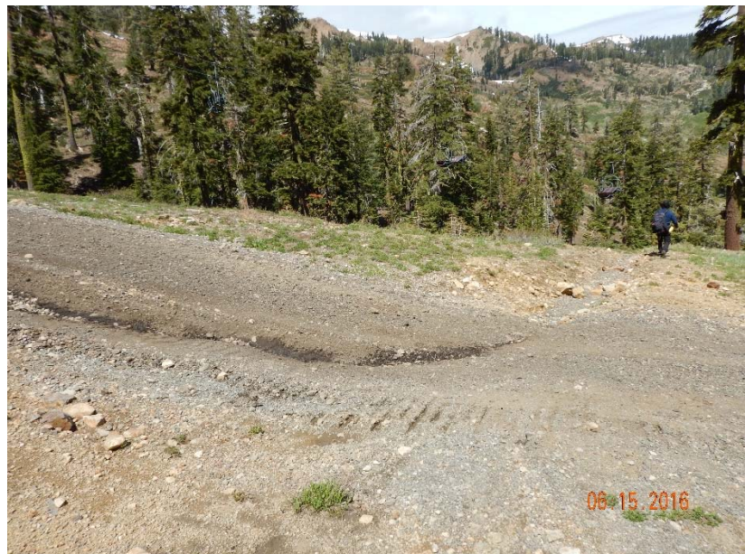
Figure 16. Riling creating inside ditch on outslope road. Rolling dip transporting larger than normal runoff off road. Outlet is being scoured and incised due to large amount of flow.
