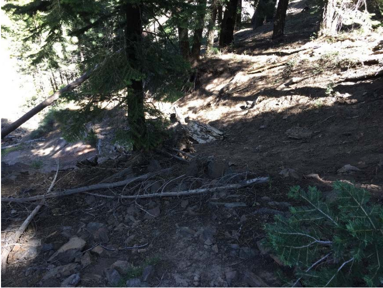
2.19: On private property. Fillslope is failing and exposing bare soils.
