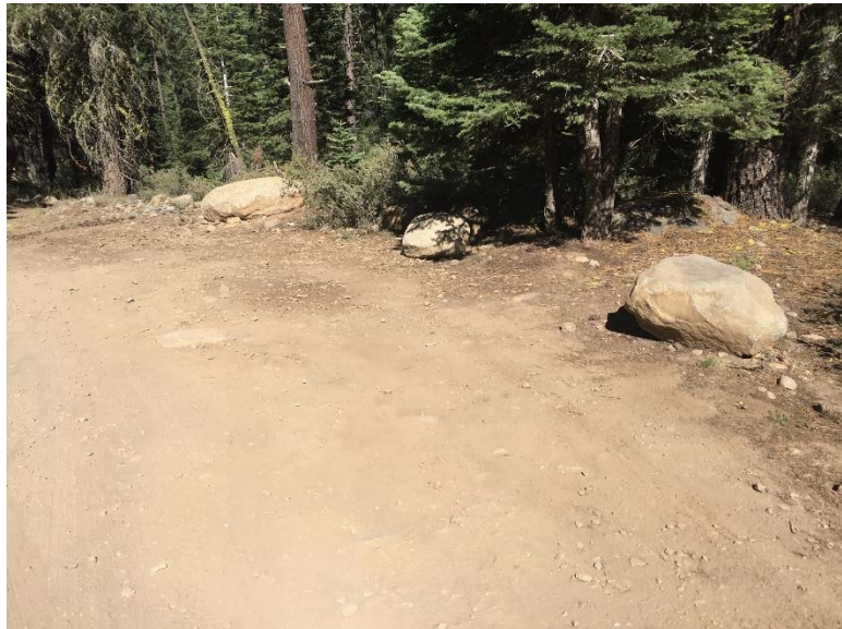
J16: Failed waterbars here allow for runoff from J6 to continue down to road and accumulate more surface runoff. The leadout here still captures some runoff of J6 and is filled with sediment. Sediment continues into Jackass Creek.
