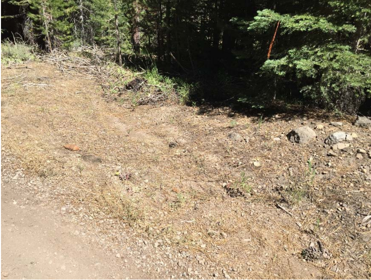
J22. Leadout filled with sediment from runoff of J10. Sediment continues into a meadow.
