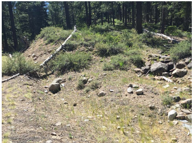
2.18: On private property. Leadout is catching excessive amounts of runoff from the upslope portion of road. Incision at the outlet of the leadout and fillslope occurs.
