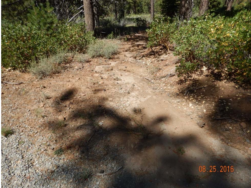
Leadout from road that has collected large amounts of sediment.
