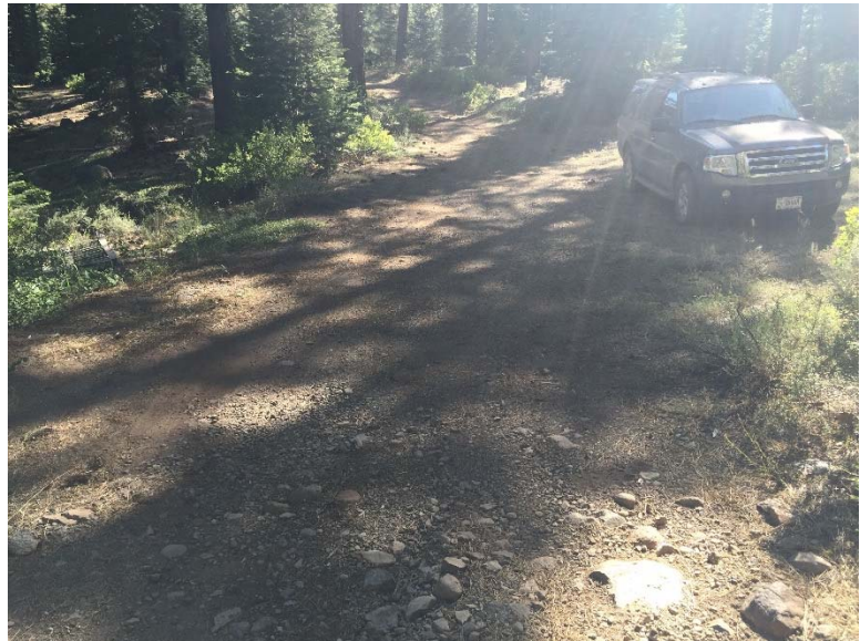
J18: Road begins to outslope before reaching crossing J19: Runoff from J6 leaves road before passing over culvert and enters Jackass Creek.
