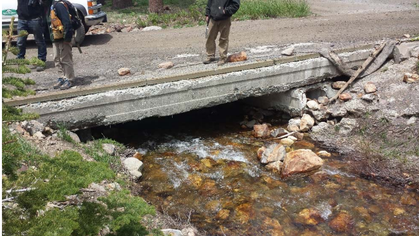
Figure 6. Bridge crossing over perennial channel. Straw waddles installed to prevent water from flowing over the top of the bridge and into the channel have failed.
