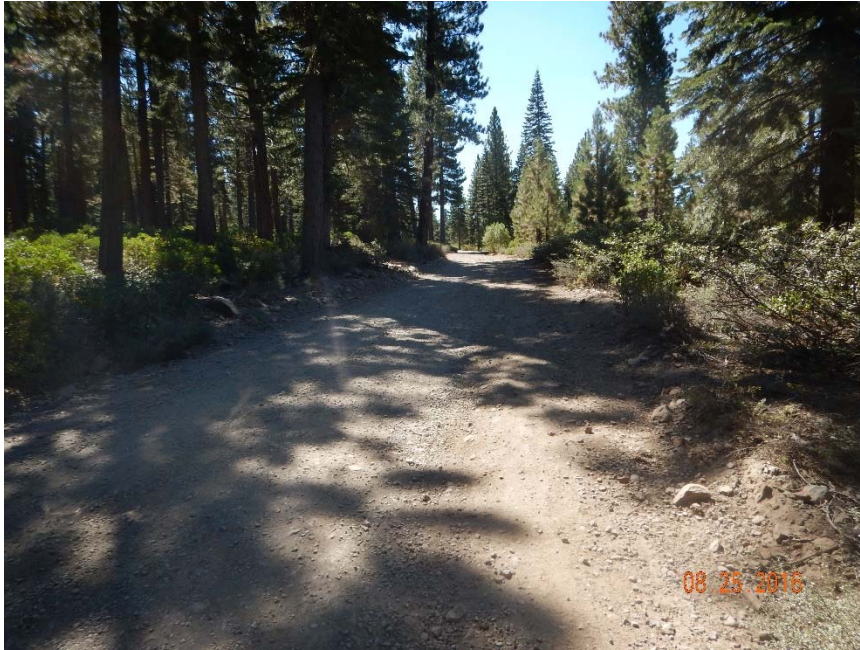
Looking down main Sawtooth 06 road with gravel road surface. The 06 road mainly consists of gravel road surfaces.
