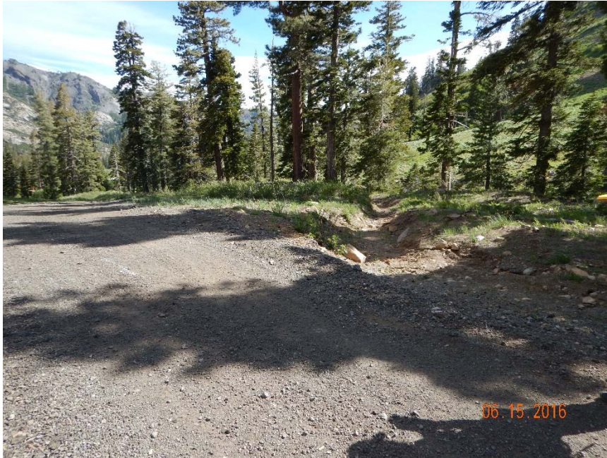
Figure 1. Leadout incision from large amounts of discharge flowing onto road from adjacent hillslope. Discharge is large enough that it flows out of the leadout and into the nearby stream.
