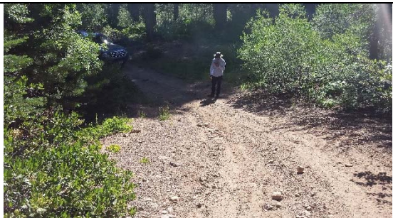
Photo 6b Heading: 180 Access road channels and main road channels converge at this point. Main channel is moderately rilled and eroded at this point.
