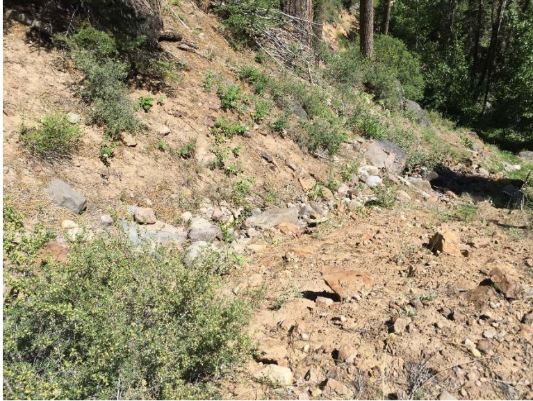
2.15: Gully is forming in inside ditch.
