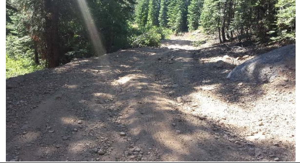
Photo 7b Heading: 135 Road is eroding as well. It is rilled and rutted. Size of transported clasts can be seen in photo.
