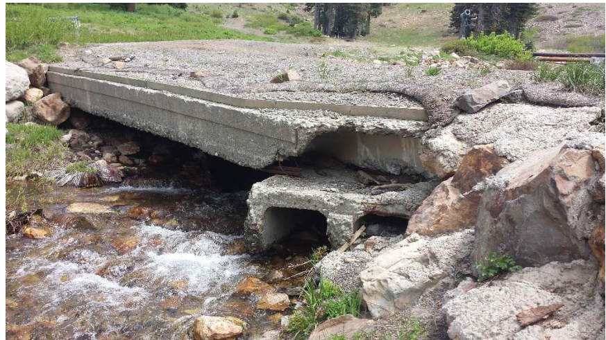
Figure 7. Bridge crossing over perennial channel. Straw waddles installed to prevent water from flowing over the top of the bridge and into the channel have failed.
