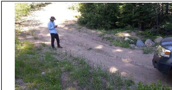
Photo 6a Heading: 285 Access road channels and main road channels converge at this point. Velocity of flow is evidenced by size of boulders in drainage (right side of photo).
