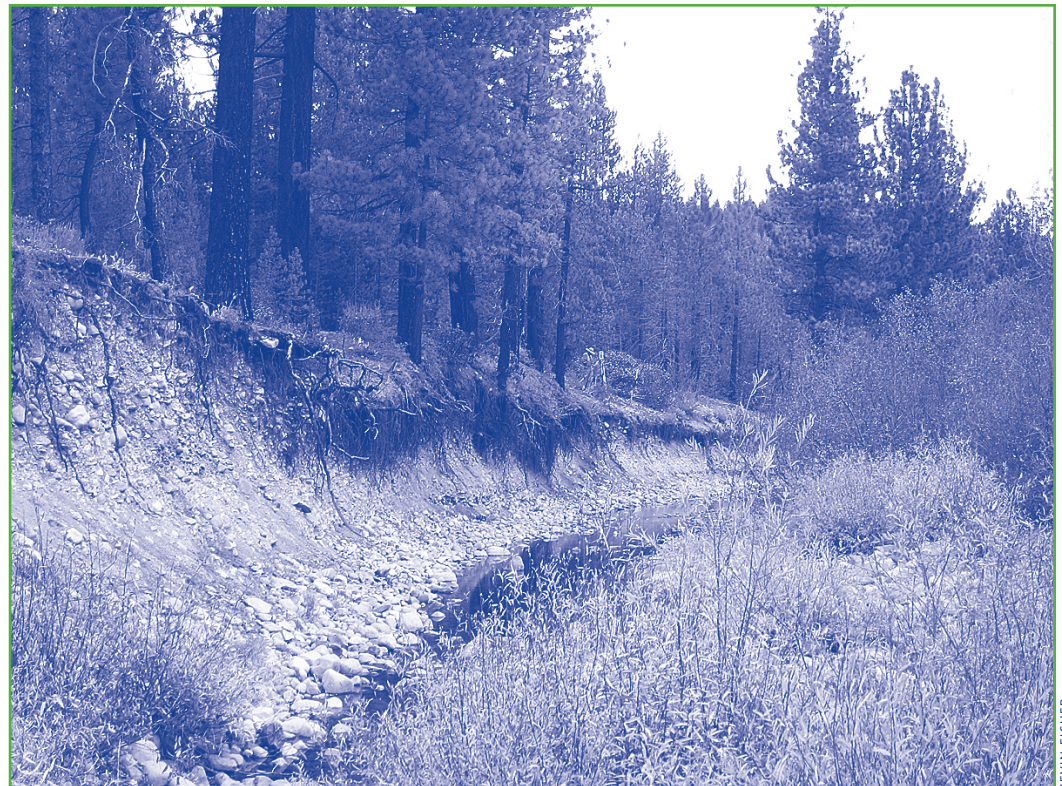
Coldstream Canyon: Typical eroding bank in the project area. Restoration will reduce erosion in the project area and the amount of sediment reaching the Truckee River.
