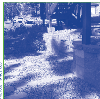
In the same yard after river-friendly landscaping, exposed soil is protected by gravel "armoring," the surface runoff is directed to a bioretention basin so that the sediment will not reach the rivers and streams, and the erosion is stopped by a retaining wall.
