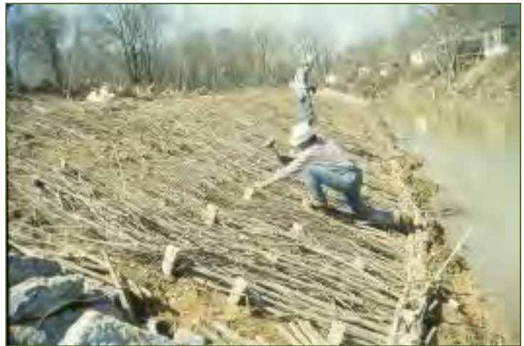
Securing a brush mattress with stakes and wire.
