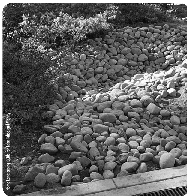
Erosion control structures like this one keep sediment from reaching waterways.
