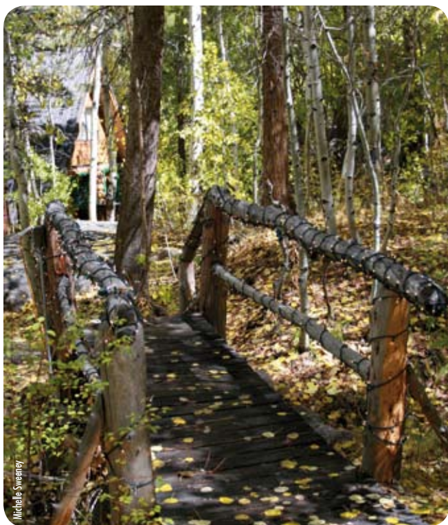
Footbridge over riparian zone
