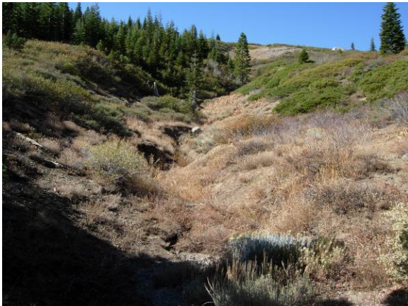
Photo 65. Looking up slope to photo 67. There is no culvert or stable crossing where this drainage intersects the road.
