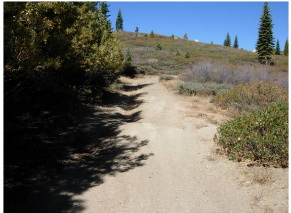
Photo 66. Roadway capture of drainage. Note that water bar directs water off road into an area that has not historically functioned as a drainage.
