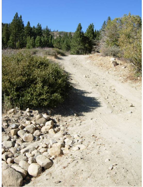
Photo 75. Main easement road. Note sediment deposited at water bar outlet in foreground.
