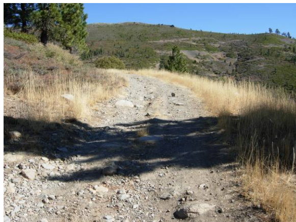
Figure 3-8. Road capture of surface flow.
