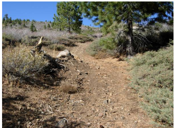
Photo 73. Old logging road exhibiting signs of erosion.
