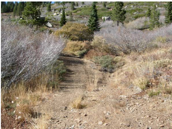
Photo 72. Gully on road formed by captured drainage.
