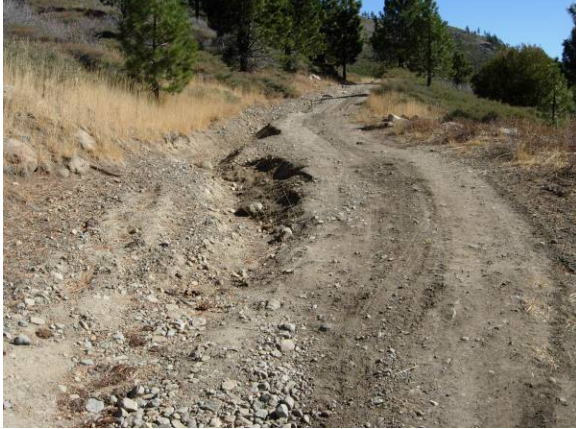
Photo 60. Looking up north road at gully created by road capture of water.
