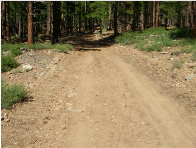
After road grading
