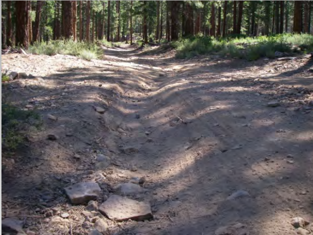
Before road grading
