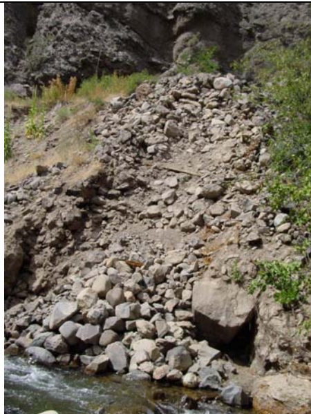
Photo 2-4. Typical example of small bank failure of coarse material in Reach MF-1.
