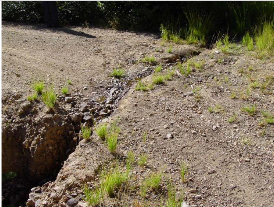
Photo 2-12. Close up of road erosion caused by small drainage just downslope of Murphy Meadows in West Fork subwatershed.
