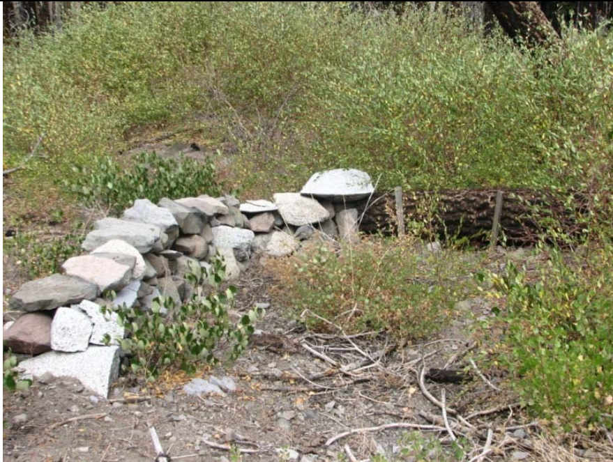
Photo 4-23. Erosion control structure in severely burned forest, West Fork Reach 2 (WF-2).
