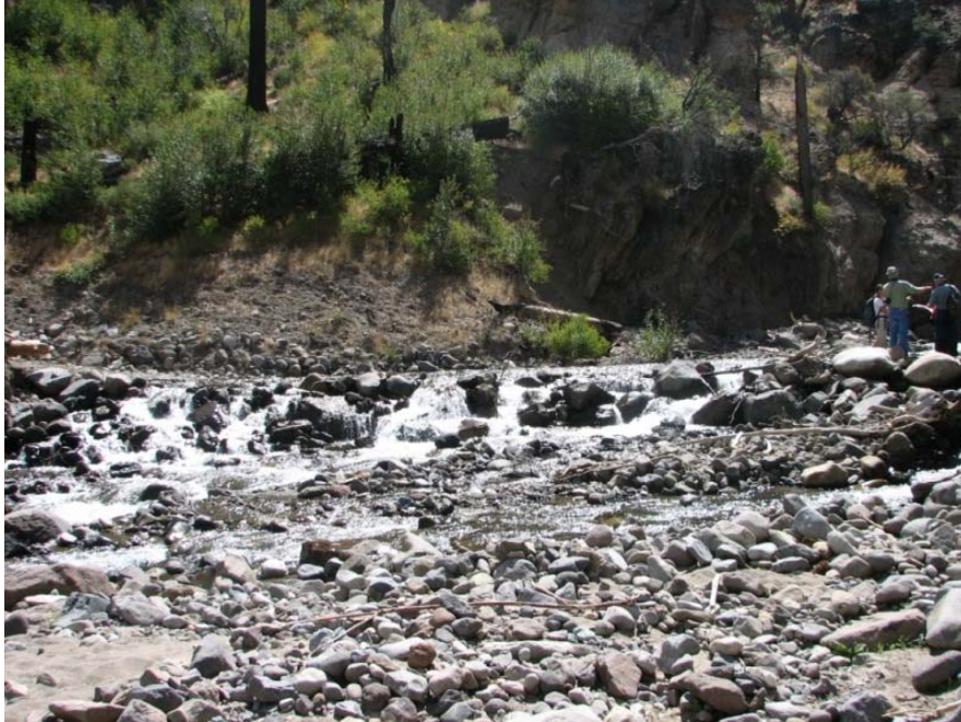
Photo 4-5. View looking upstream at a step in the channel created by road crossing, Main Stem Reach 1 (MF-1)
