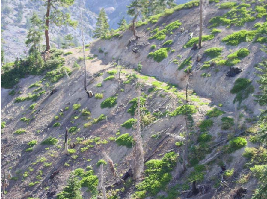
Photo 2-13. Severe erosion along abandoned road cut in West Fork subwatershed.
