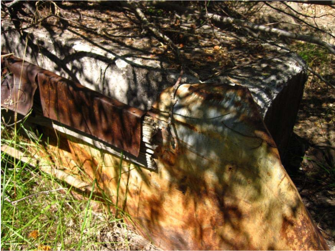
Abandoned diversion structure, Mainstem Martis Creek, Reach 1
