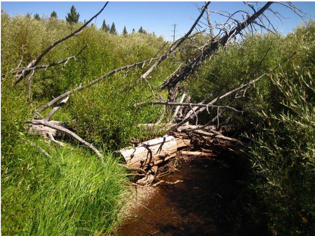
Abandoned point of diversion to irrigation ditch, Mainstem Martis Creek, Reach 1
