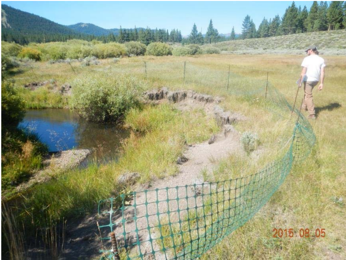
Active bank erosion, Mainstem Martis Creek, Reach 3
