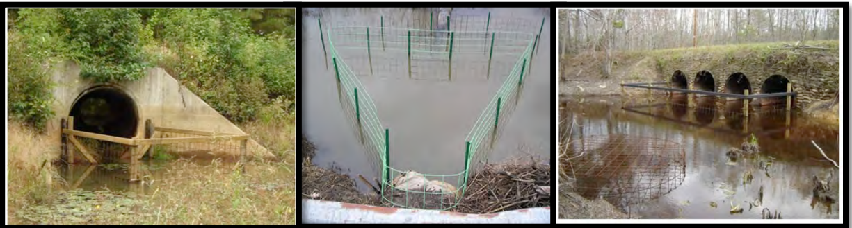
Figure 43: Examples of culvert-protective fences. From left to right: (a) and (b) are stand-alone culvert-protective fences, while (c) is a stand-alone fence combined with a flexible pond leveler pipe (underwater and not visible) and a cylindrical wire mesh cage, which provides extra protection against obstruction. Figures from Boyle (2006).
