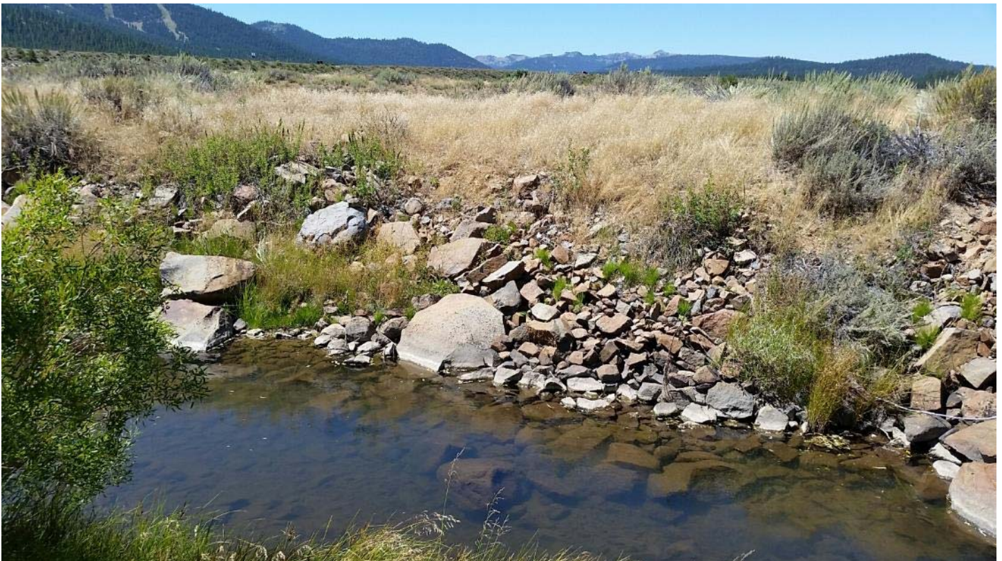
Levee, Mainstem Martis Creek, Reach 6
