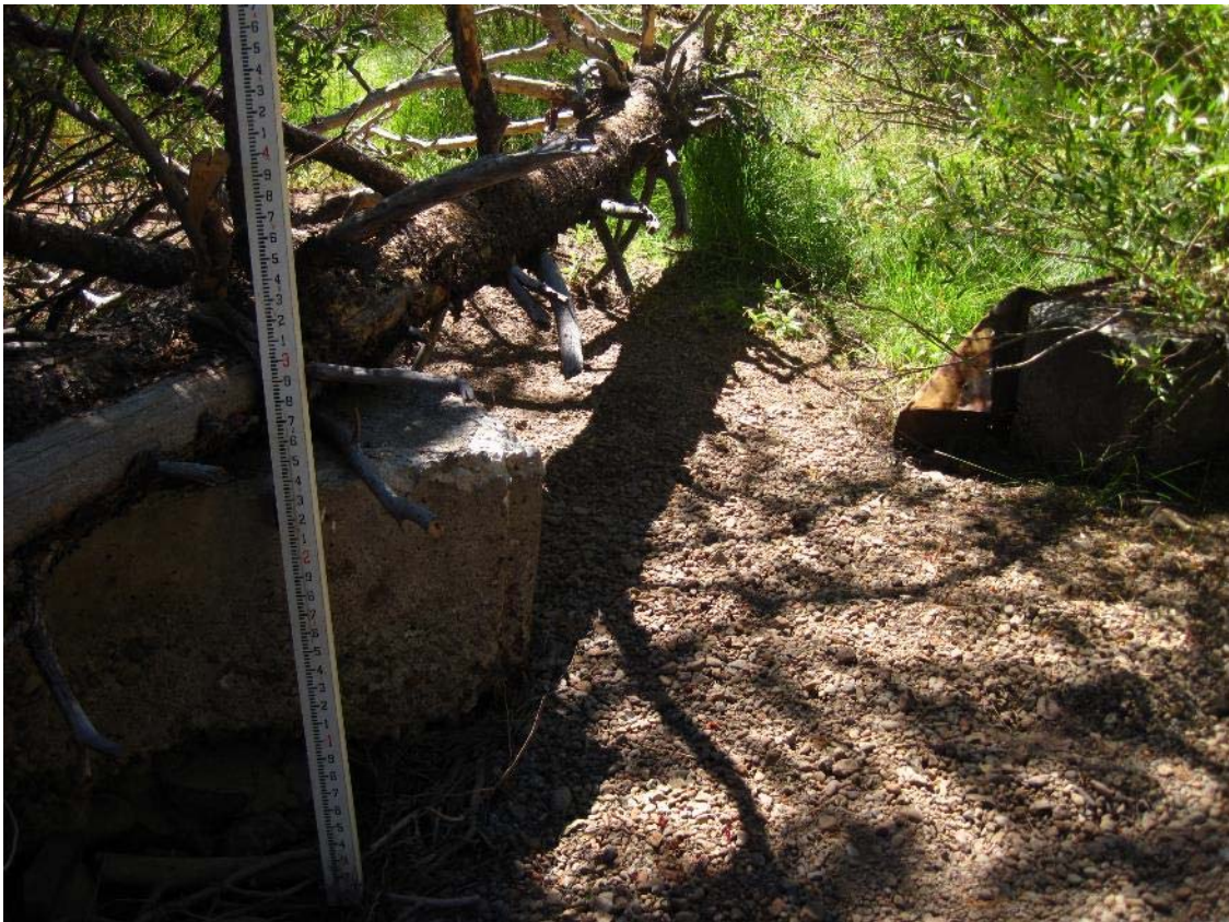
Abandoned diversion structure, Mainstem Martis Creek, Reach 1
