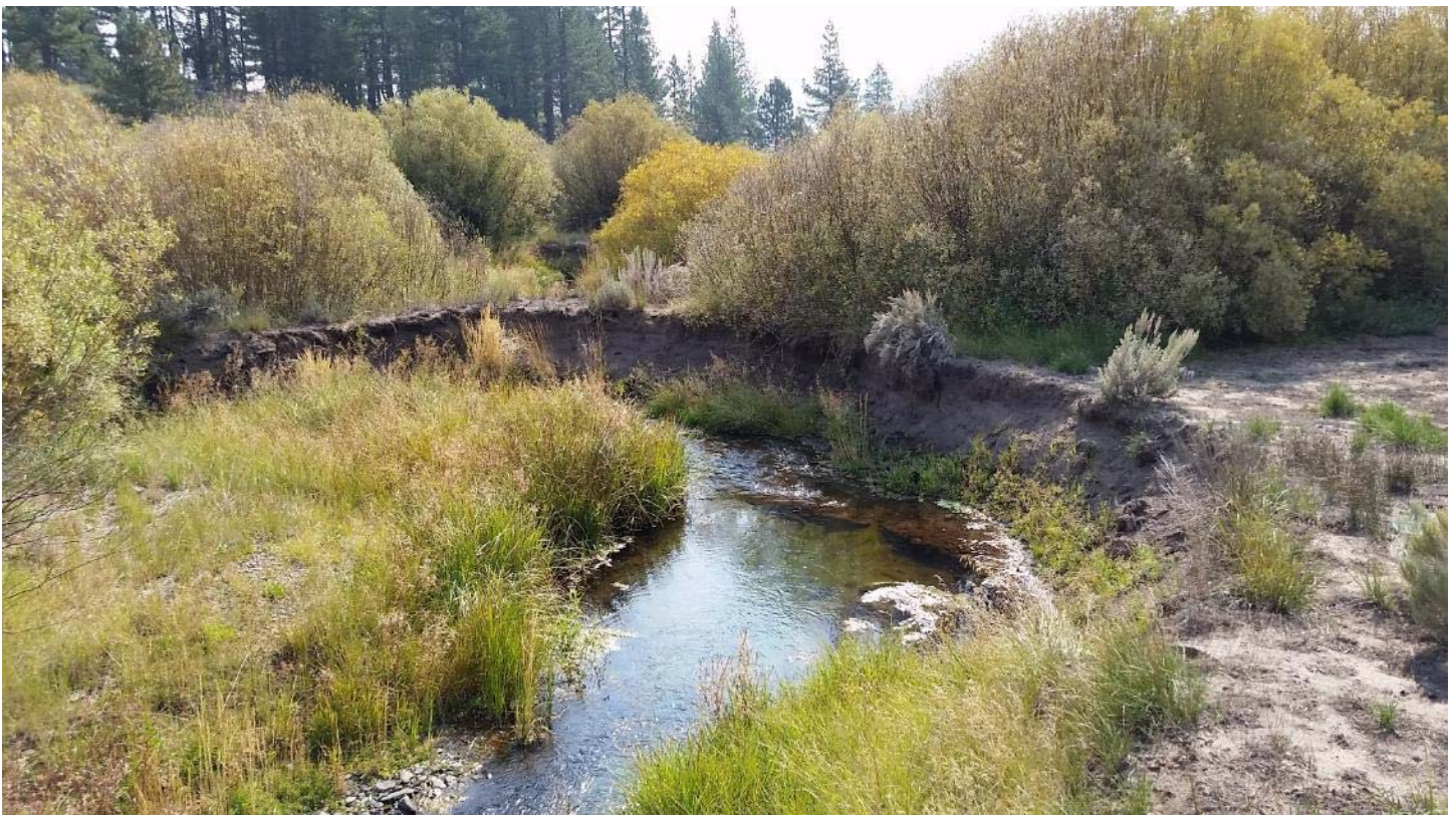
Incised channel and bank erosion, Mainstem Martis Creek, Reach 1
